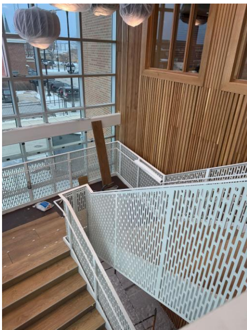
Flooring being installed on new staircase.
