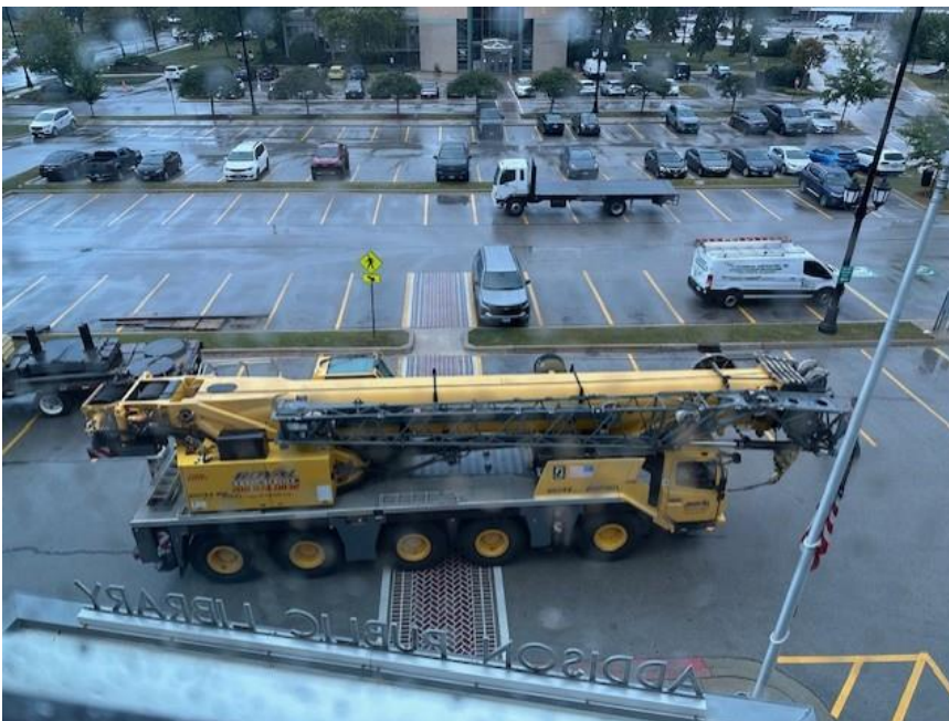
Crane delivering and removing hvac parts to the roof.
