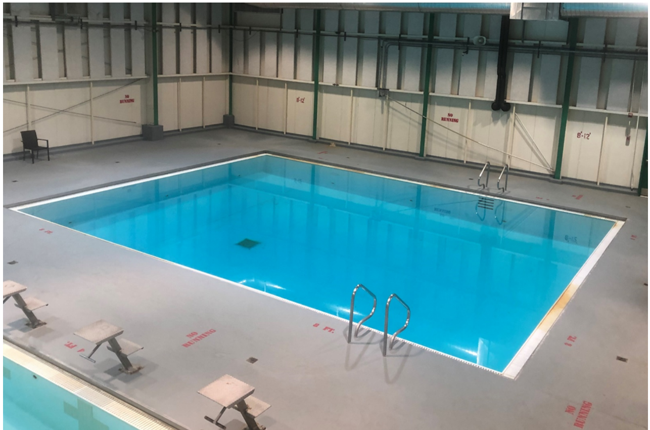
Former Dive Well – looking northwest
