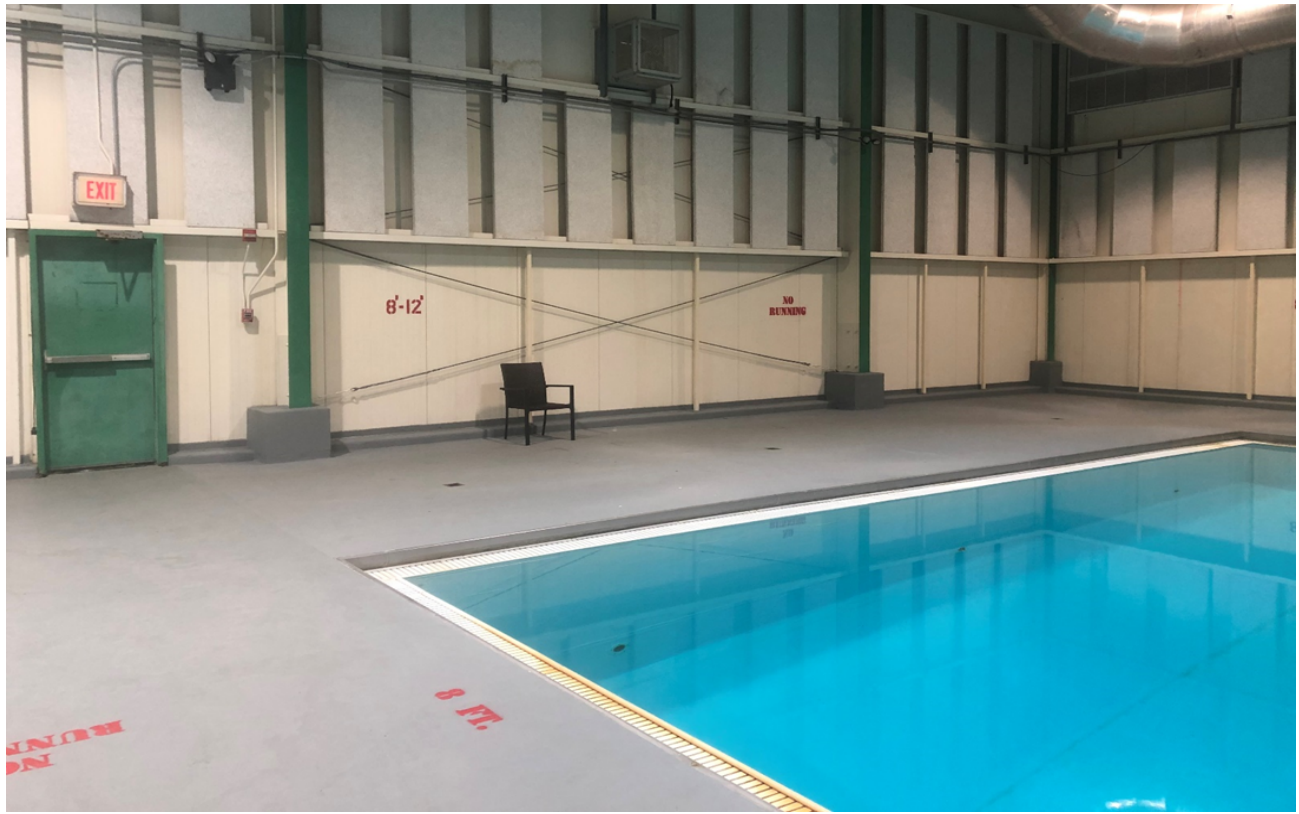
Former Dive Well – looking northwest
