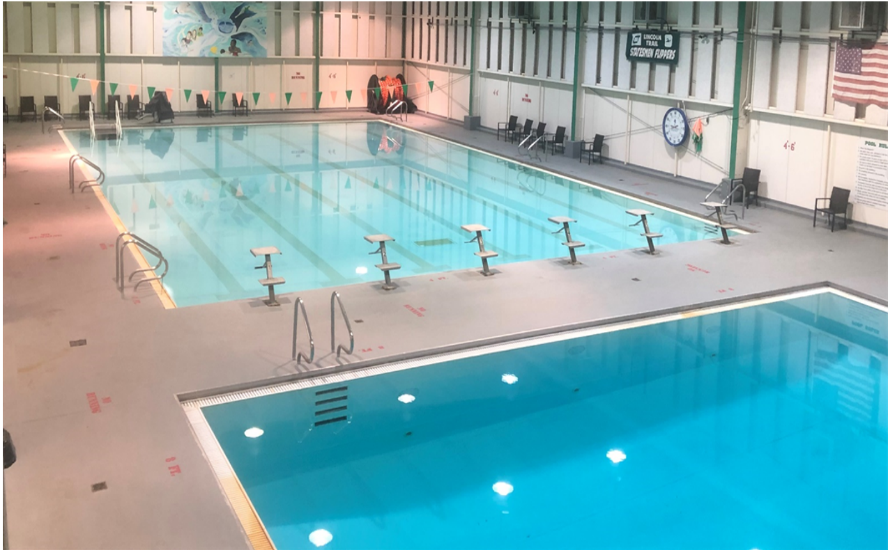
Main Pool and Former Dive Well – looking southwest
