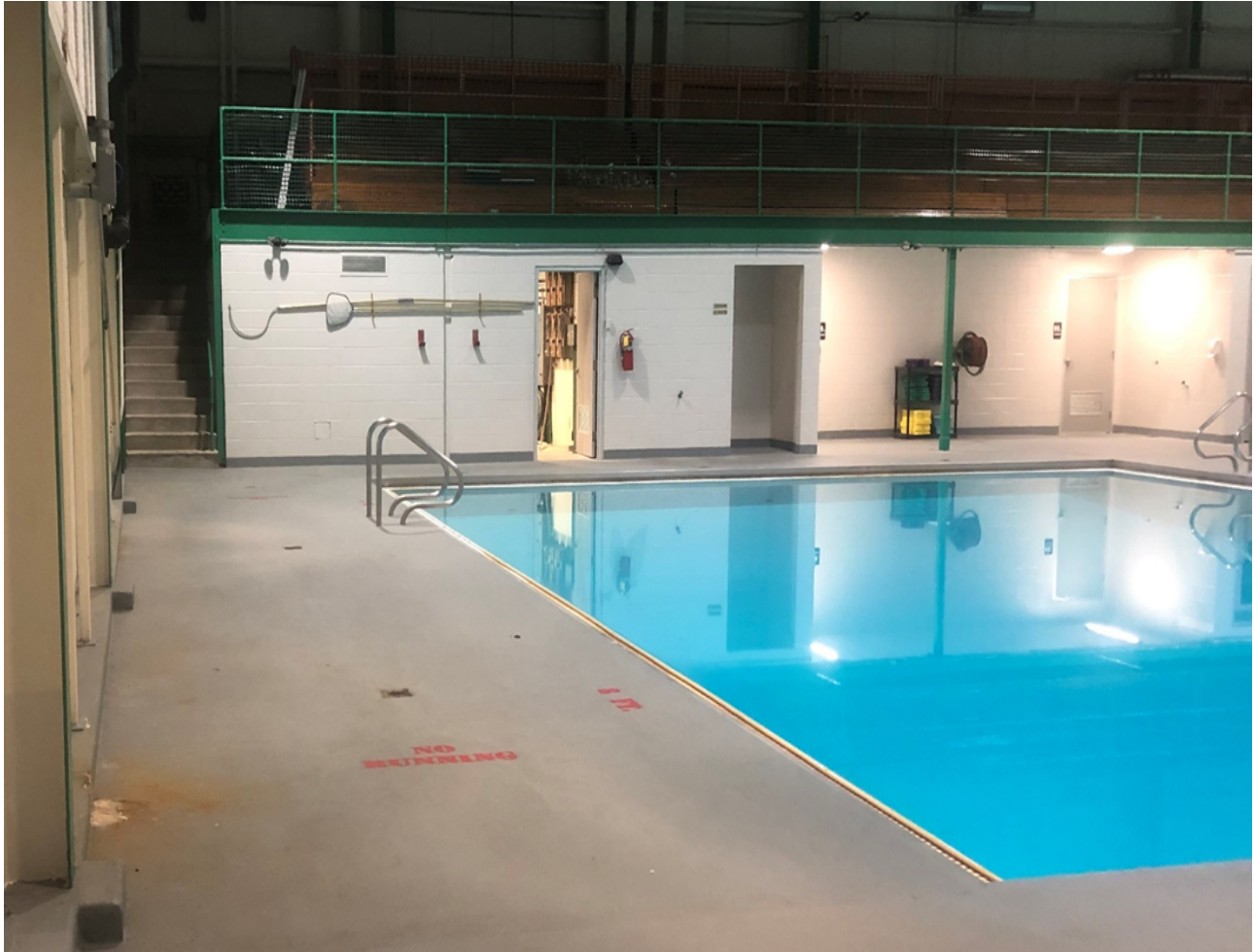
Former Dive Well – looking east
