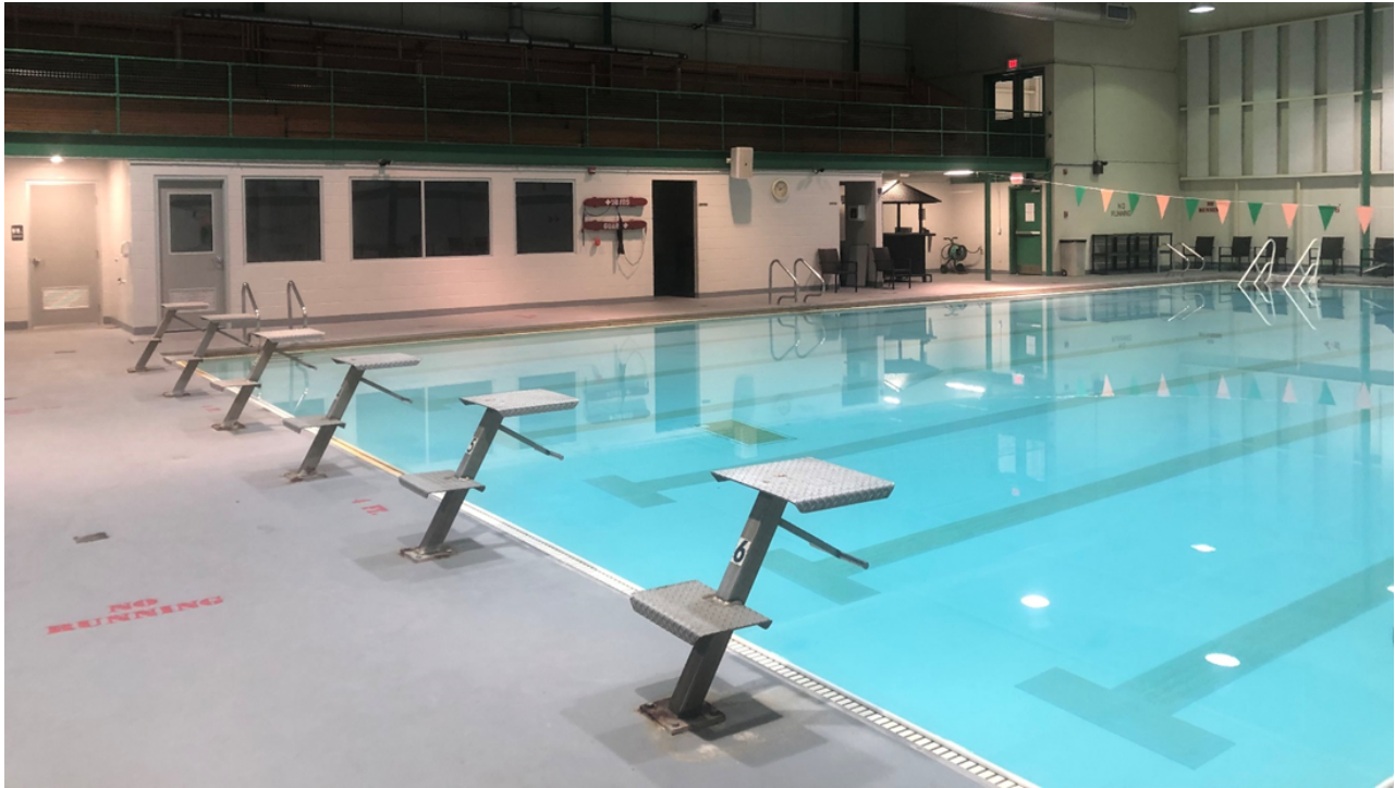
Main Pool – looking southeast
