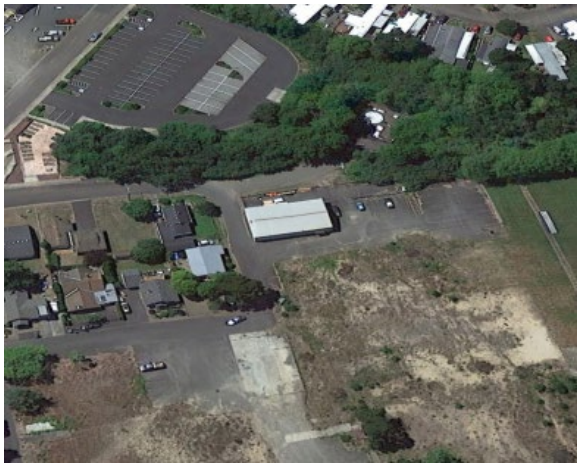
Former Facilities & Maintenance Building
