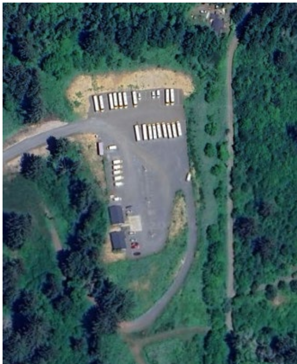
New Facilities & Maintenance Building (alongside the Bus Barn)
