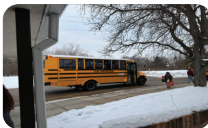
Weather Exposure: Pick-up and drop-off areas lack weather protection
