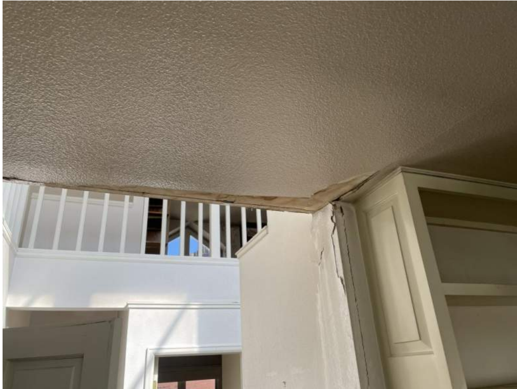
Figure 3- Damage to third floor framing at rear wall as viewed from the kitchen.
