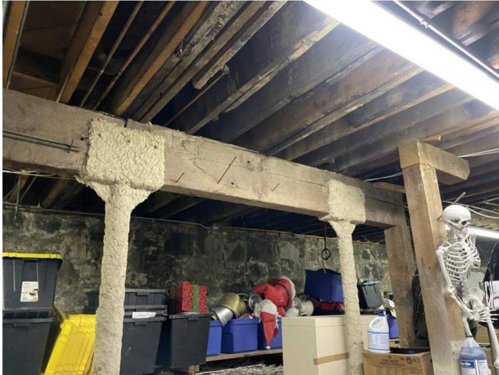
Figure 15- Upgraded framing in basement. Column locations correspond to hallway bearing walls above.
