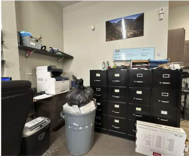
General circulation with files and furniture obstructions
