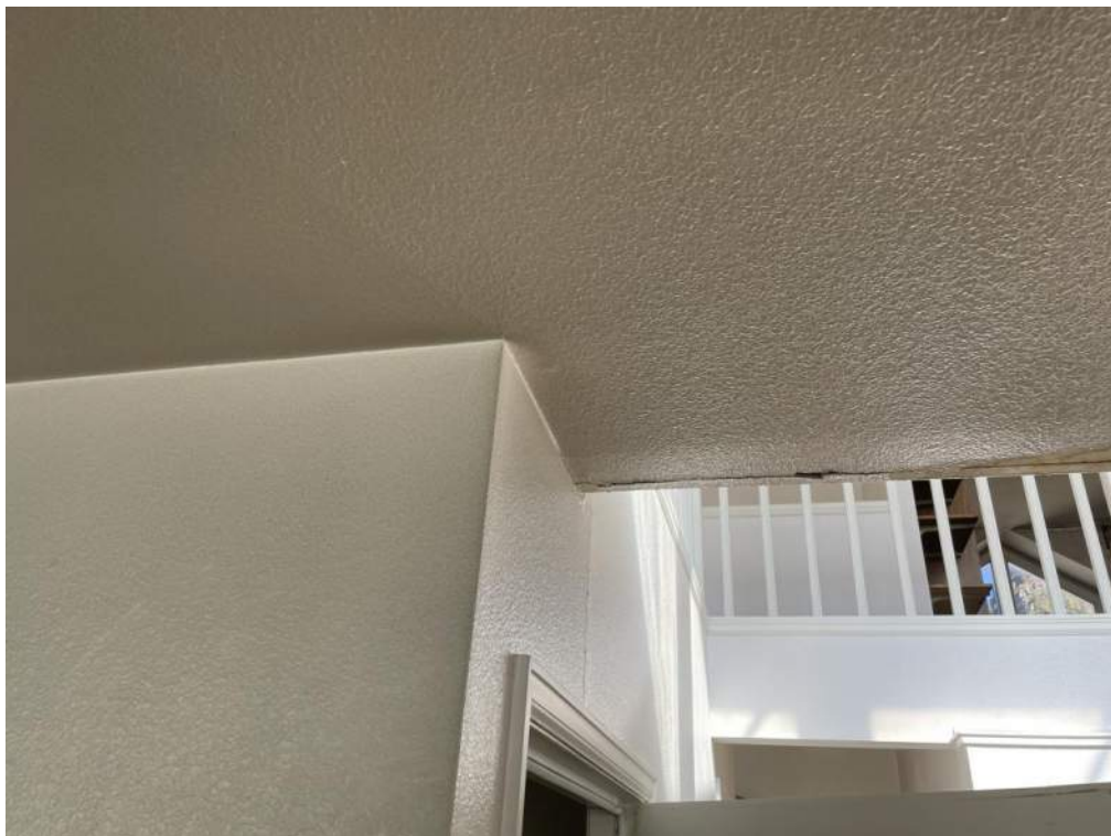
Figure 4- Damage to third floor framing at rear wall as viewed from the kitchen.
