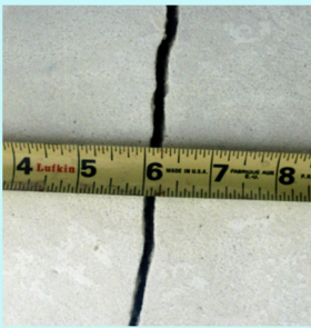
1/4" concrete crack
