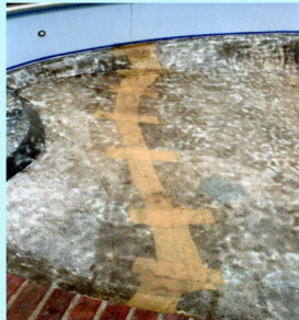
Crack repair with Kevlar (by DuPont) and special resins
