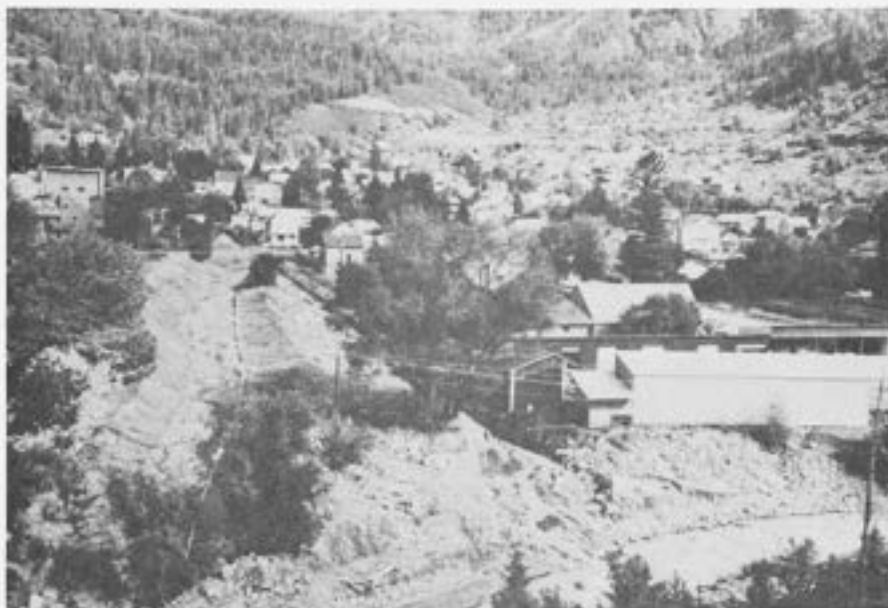
Figure 14. Portland Creek flume after 1982 event. Looking east from Oak Street. Debris is spread out where flume was broken in 1981.
