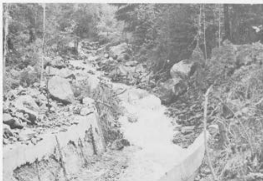
Figure 33. Cascade Creek flume entrance, 1982, before modification.
