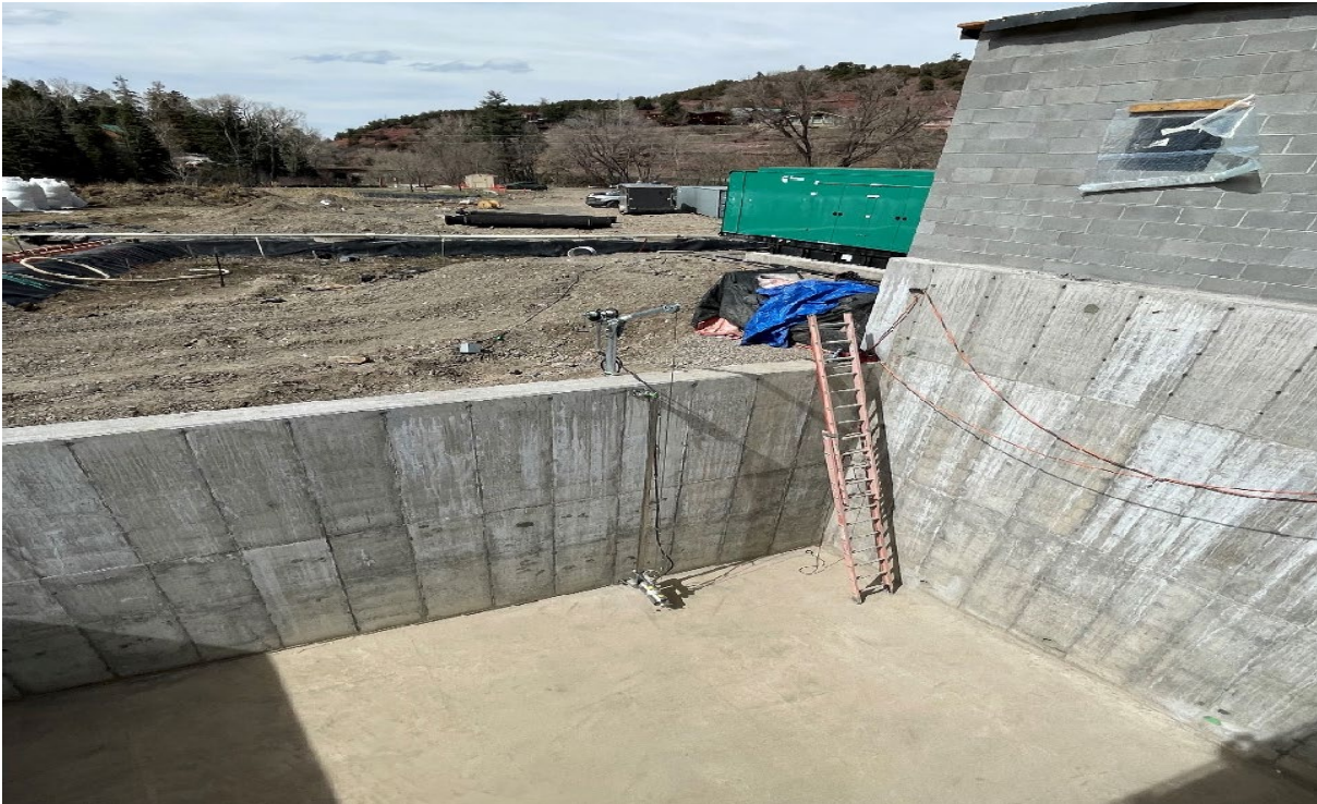
Installed mixer and davit crane in the EQ tank
