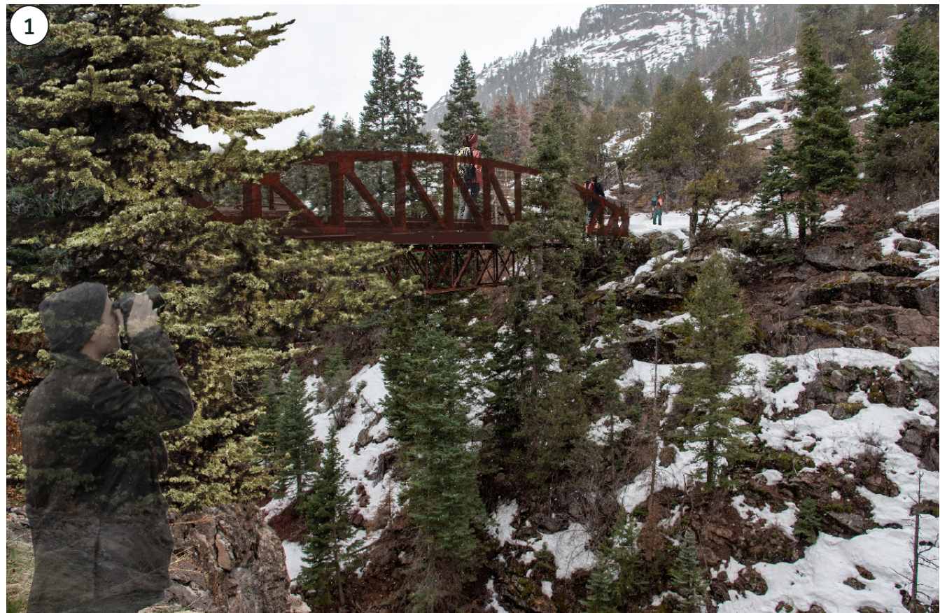
New pedestrian bridge for trail access to Box Cañon
