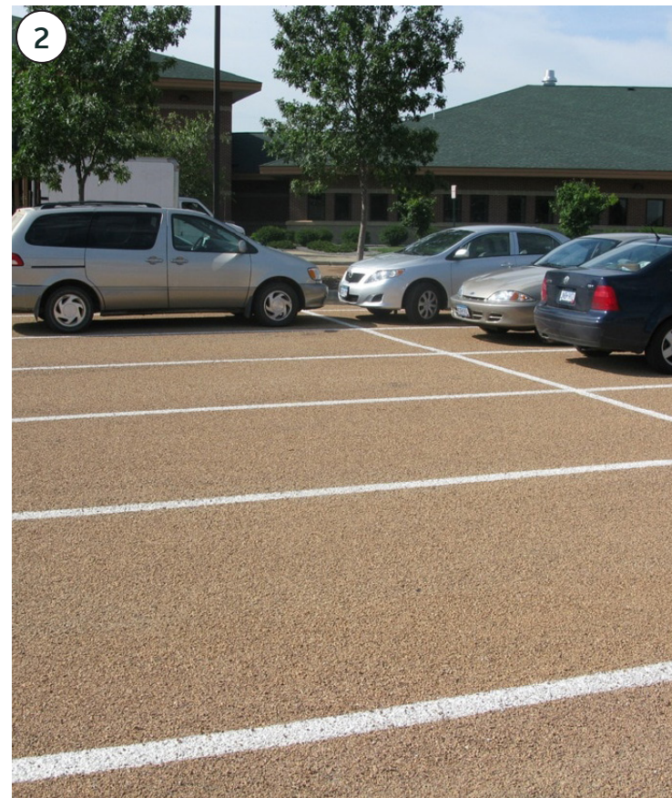
Delineate parking areas by temporary striping
