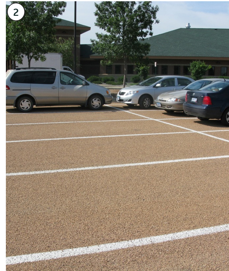
Delineate parking areas by temporary striping
