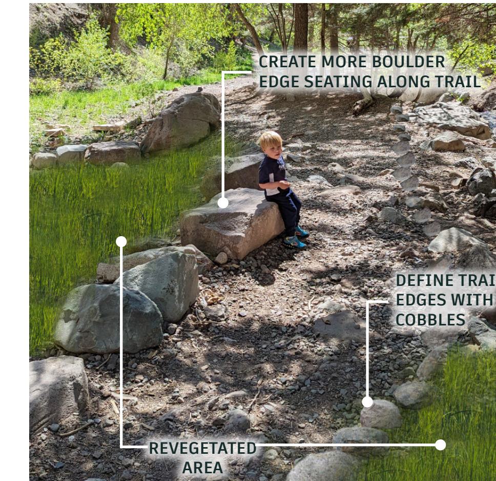
Create boulder edge seating, revegetate around trail, and define trail edges with cobbles or boulders
