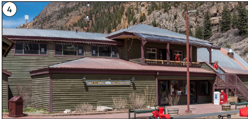
4 Bath House Analysis: Weight room on upper level needs reinforcement or new building.
