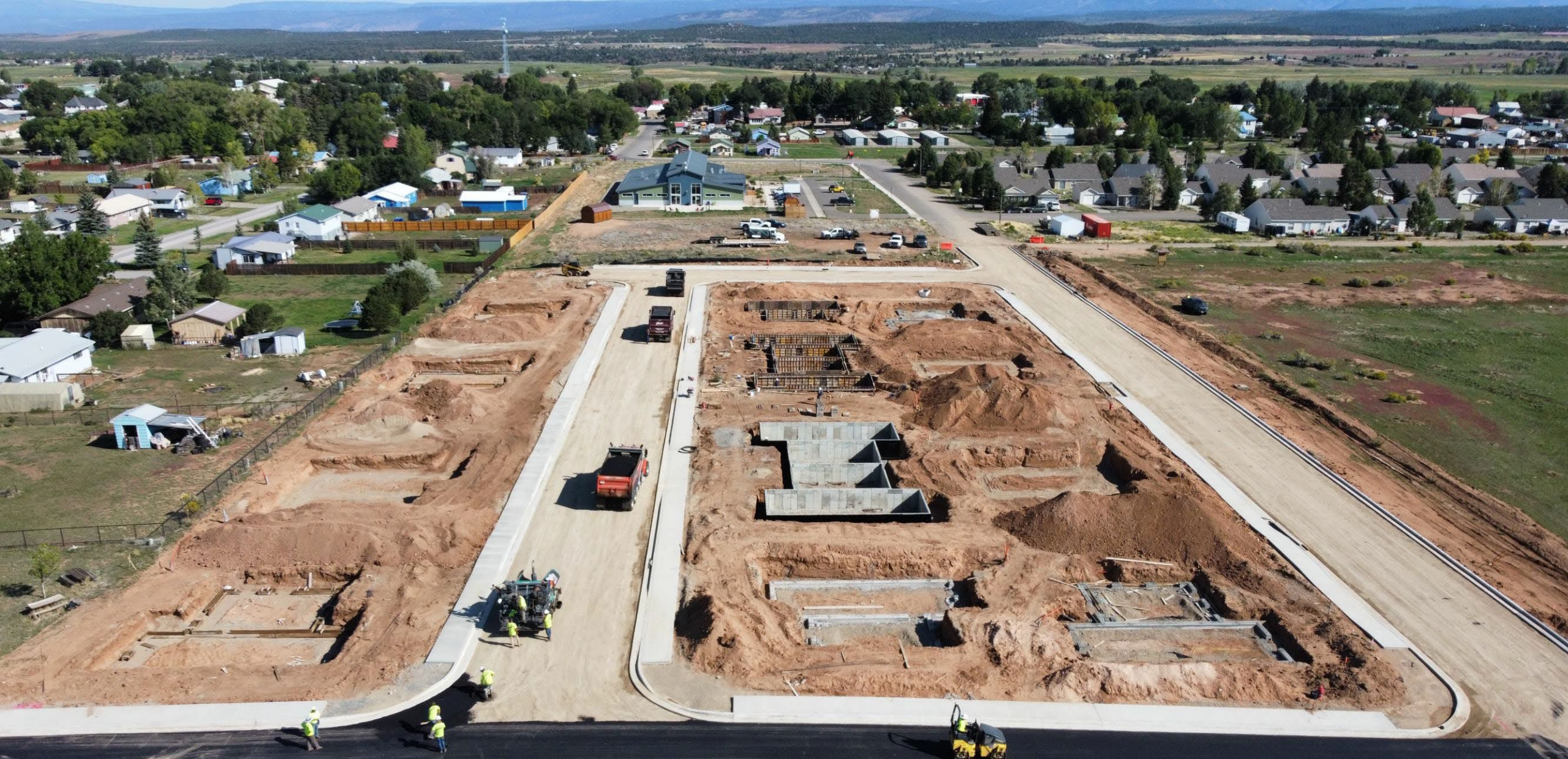
SITE INFRASTRUCTURE & UTILITIES
