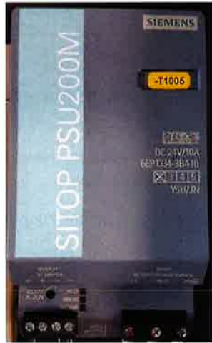
Figure 45 - READy Collector Base power supply
