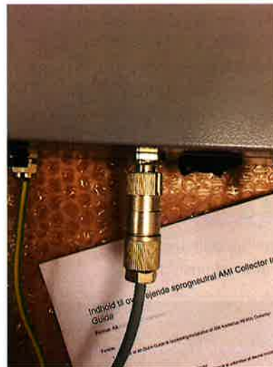
Figure 27 - Power connection installation 2
