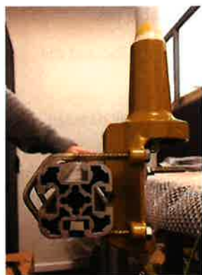
Figure 24 - Antenna installation on antenna beam
