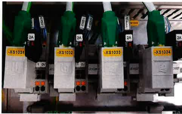
Figure 32 - READY Collector Base Ethernet connectors
