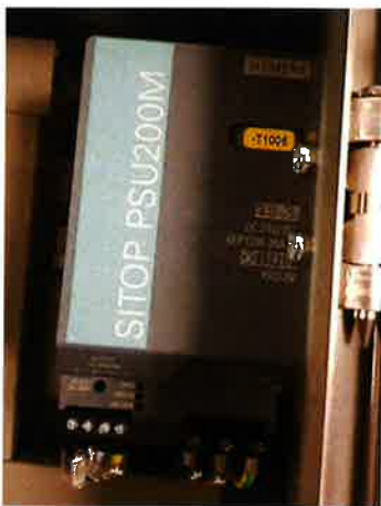
Figure 42 - READY Collector Base power supply
