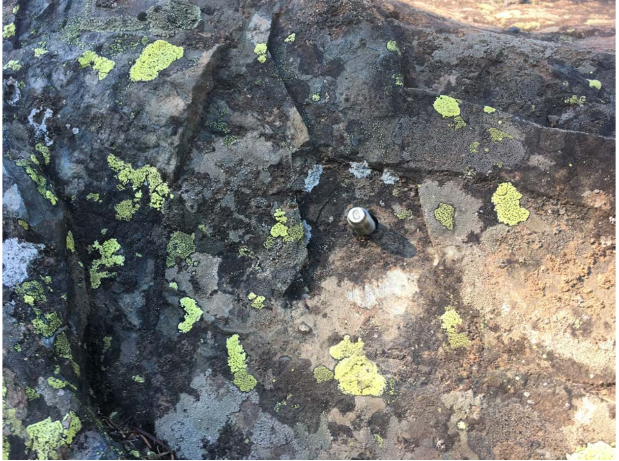
Photo: Damaged bolt on the practice course.
