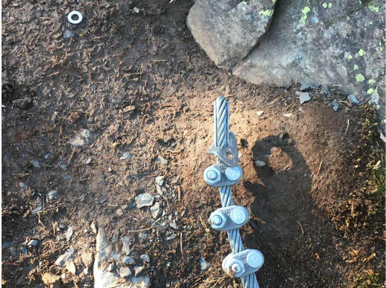
Photo: Damage to the practice course. The cable and washer were found on the ground.
