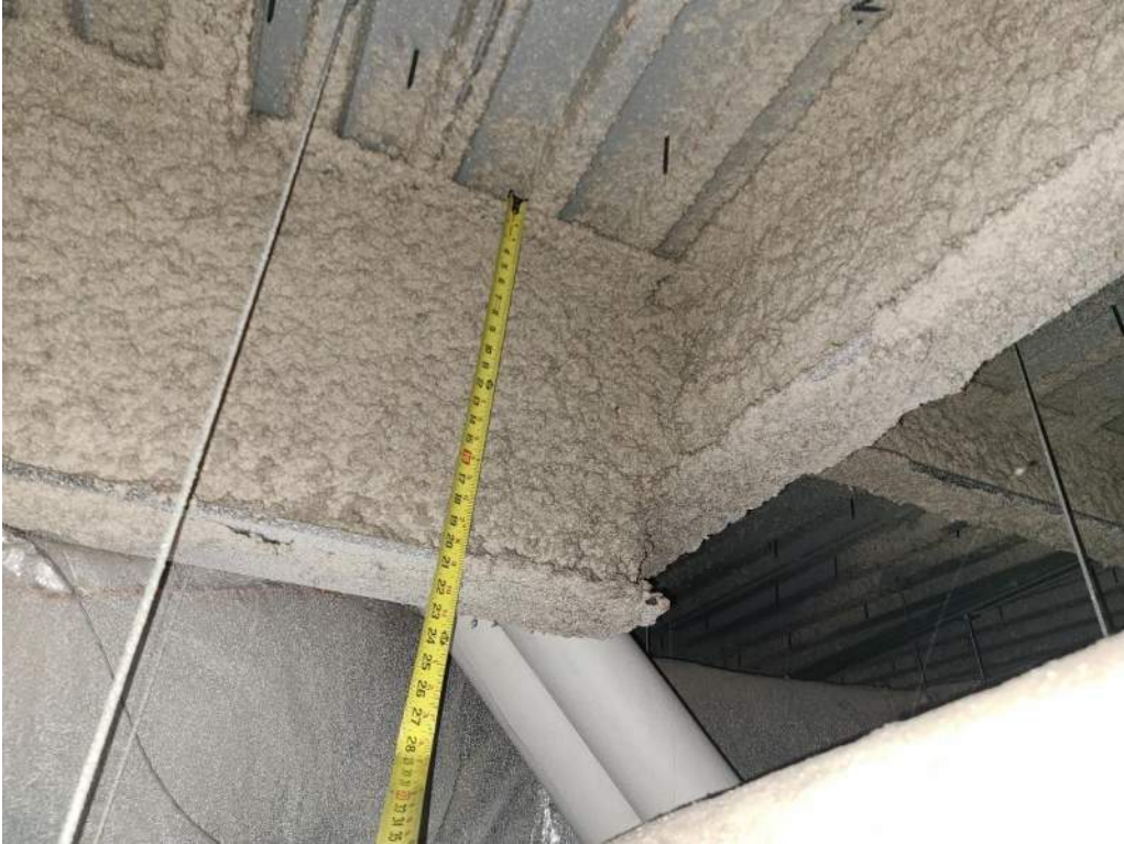
Photograph 9 – Overall View of Library Roof Framing
