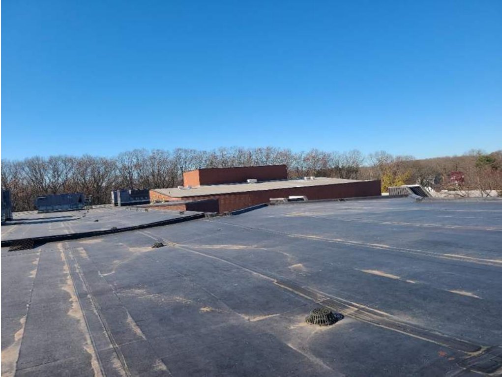
Photograph 11 – Overall View of Roofing
