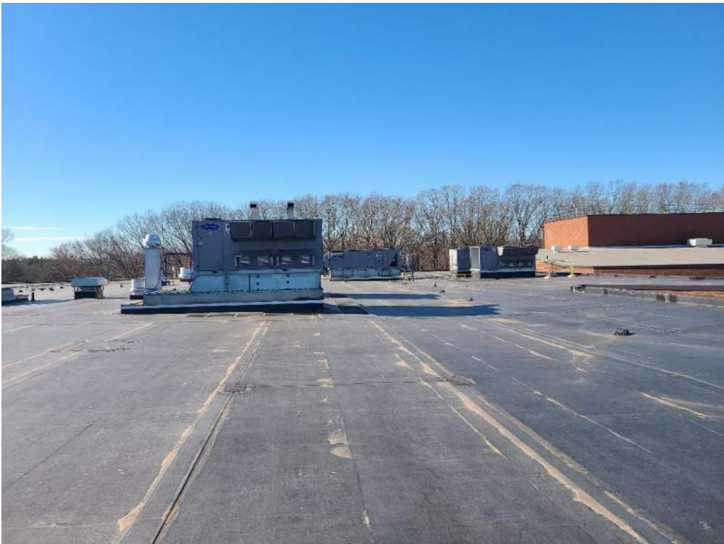
Photograph 12 – Overall View of Roofing
