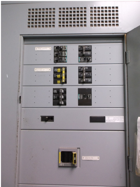
New 'Siemens' Distribution panel (DP)
