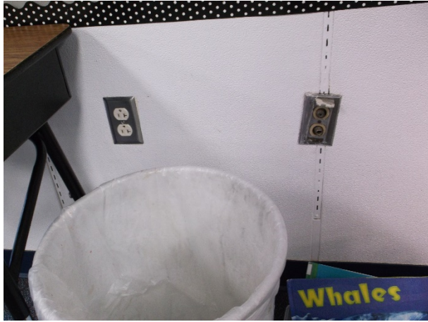
Recessed mounted receptacle
