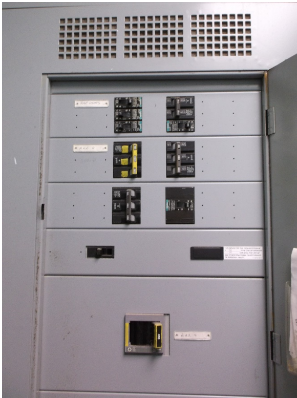
New 'Siemens' Distribution panel (DP)
