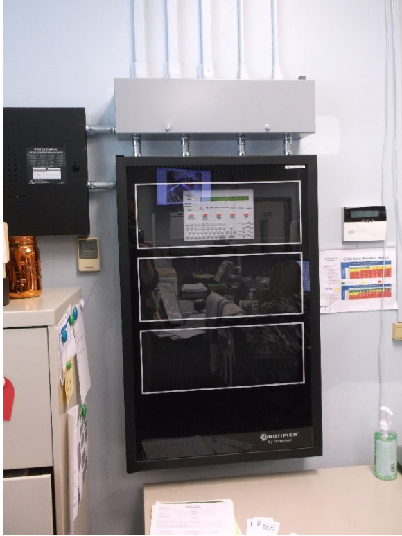
New 'Notifier' Fire alarm Control Panel in Main Office
