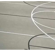
POURED GYM FLOORING
