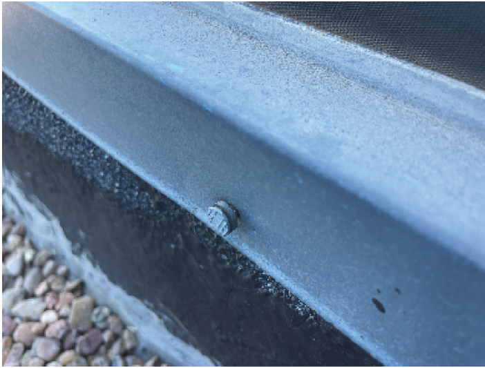
Underdriven Fastener
