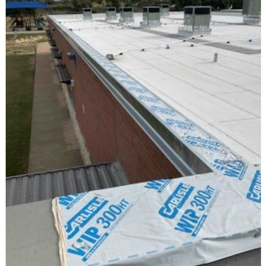
Photo: JWE Roof Trim
