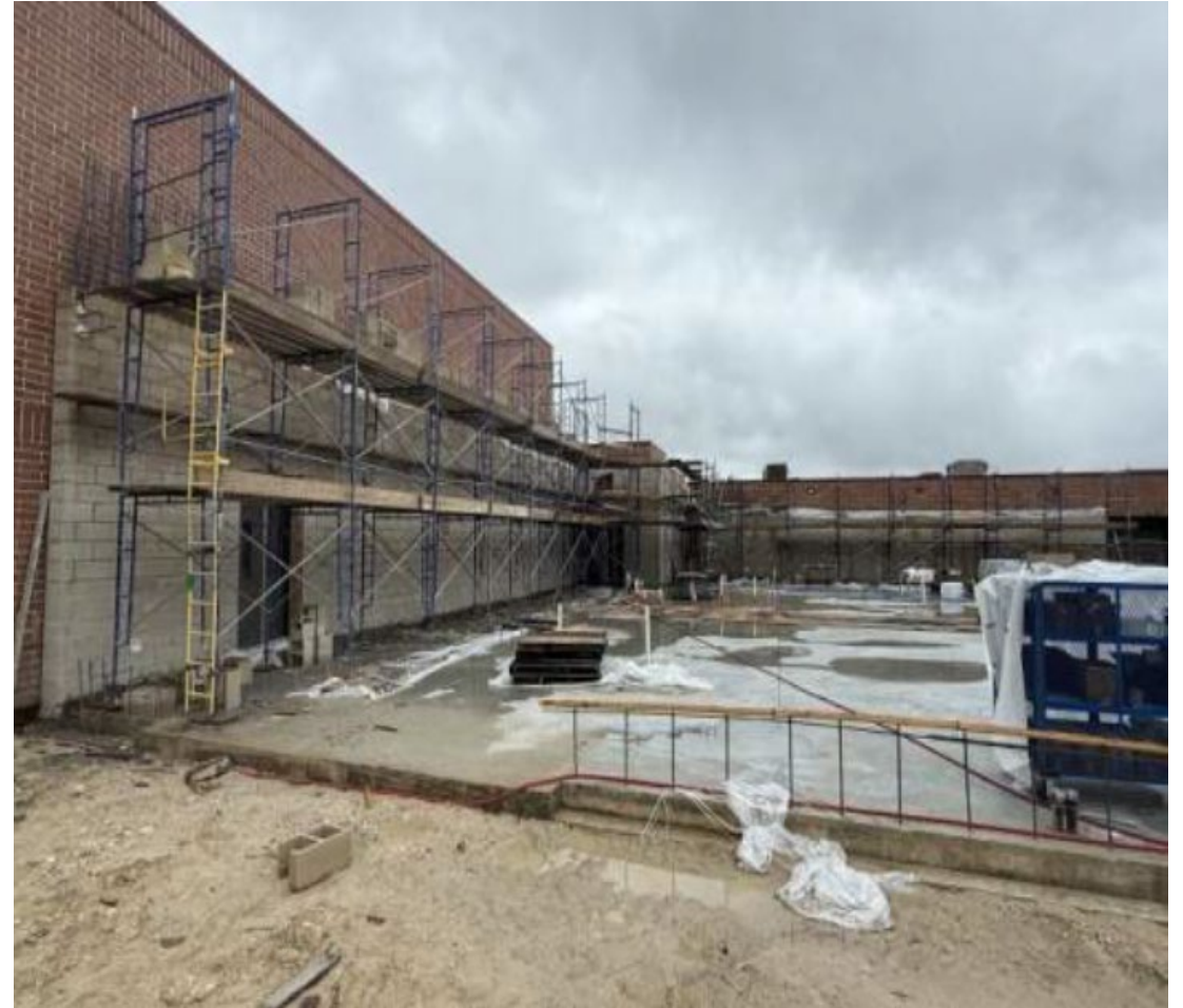
Photo: Band Hall CMU/Slab
