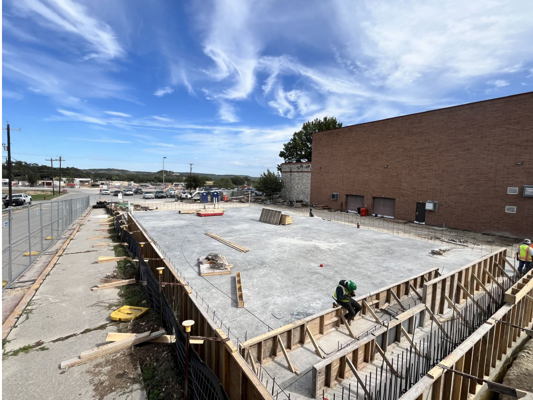
Photo: WHS Weight Room Slab Poured
