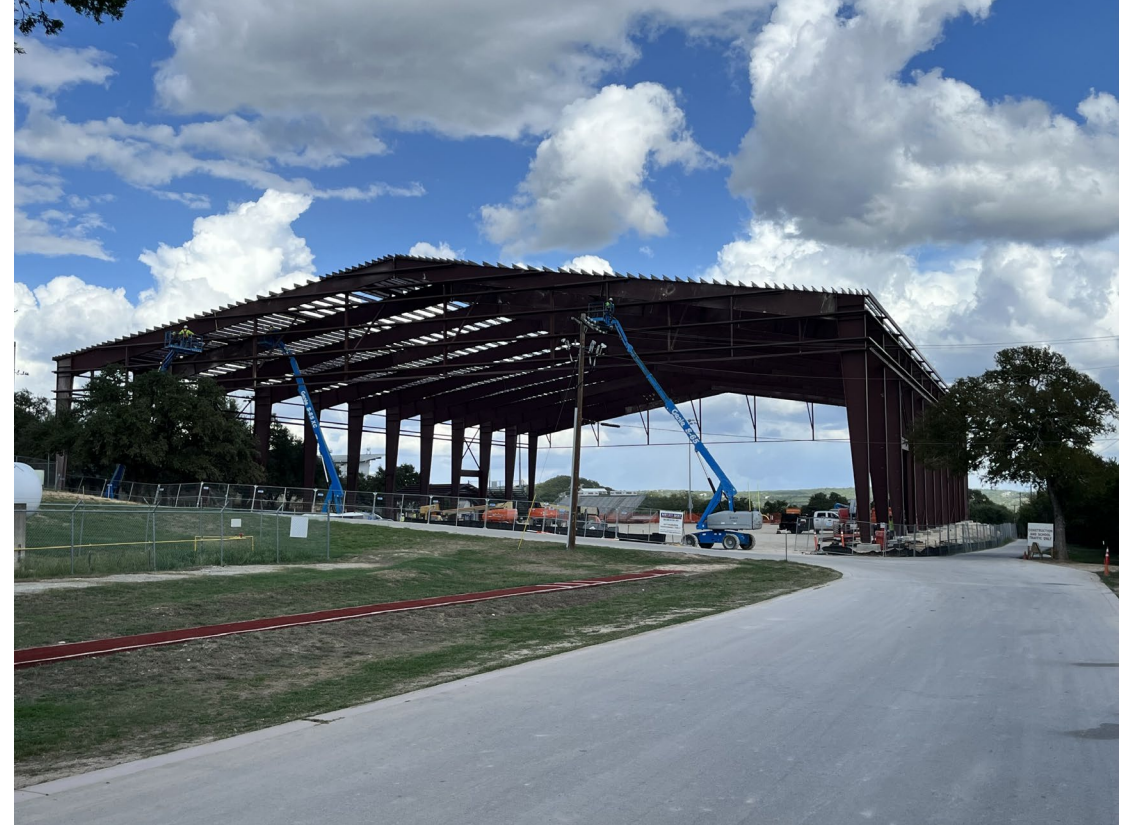
Photo: SMAC Bldg Steel
