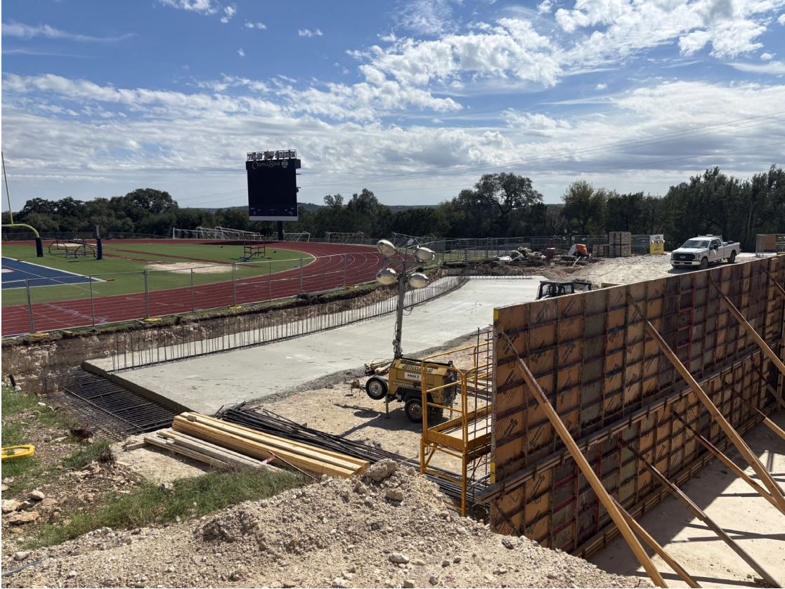
Photo: Underground Detention Pond
