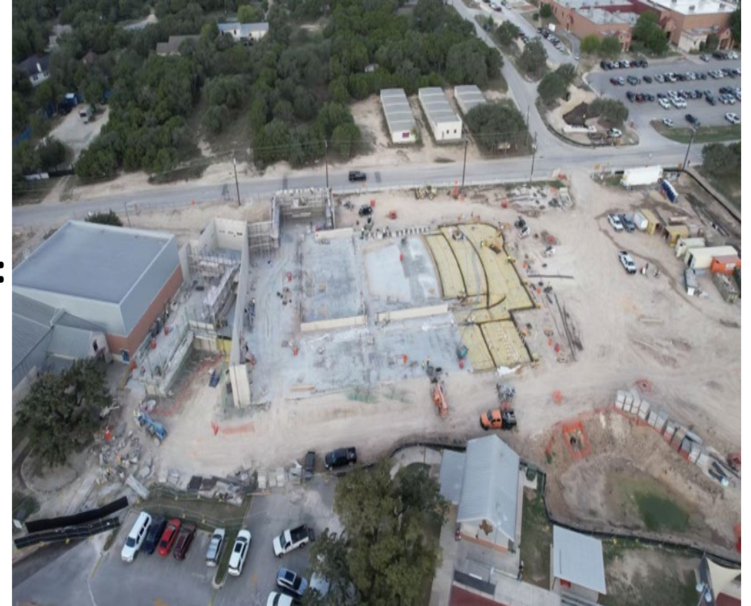
Photo: Slabs Poured @ Performing Arts
