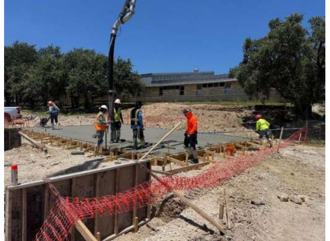
Photo: SMAC Storage Slab Poured
