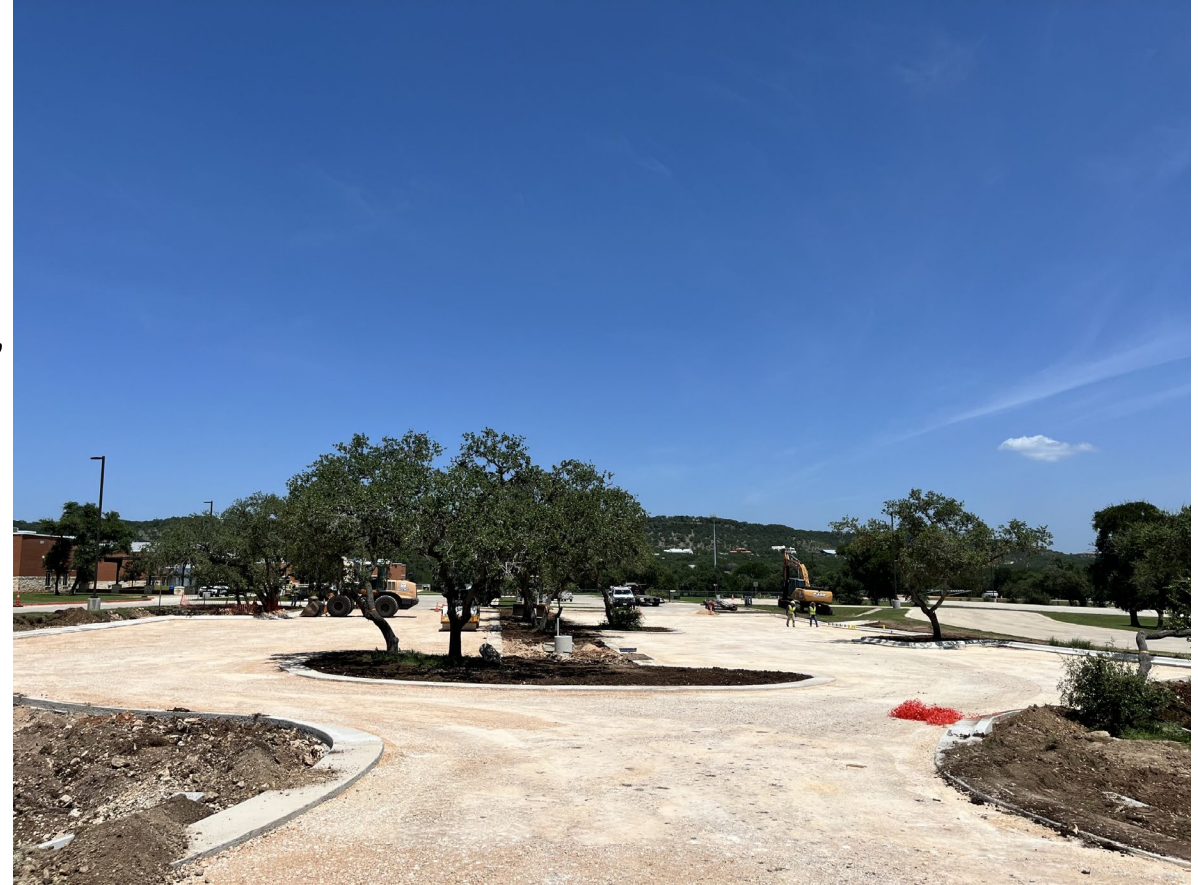
Photo: BHP New Parking Lot
