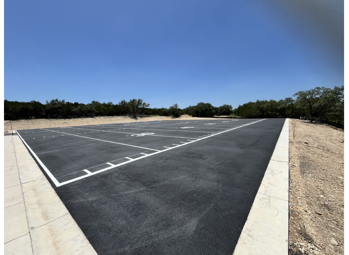
Photo: Asphalt at Band Marching Pad
