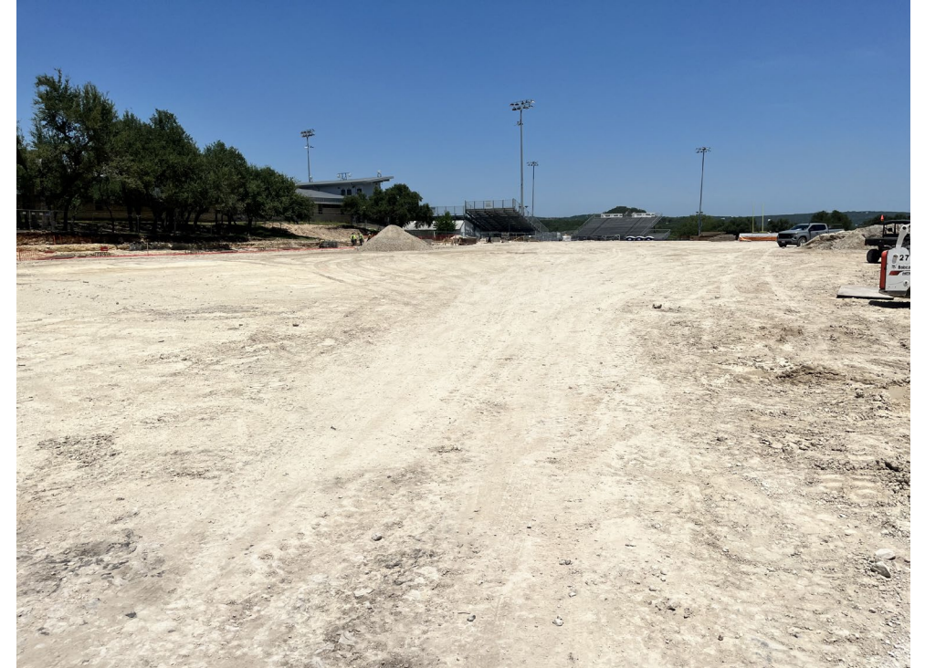
Photo: Covered Multipurpose Pad
