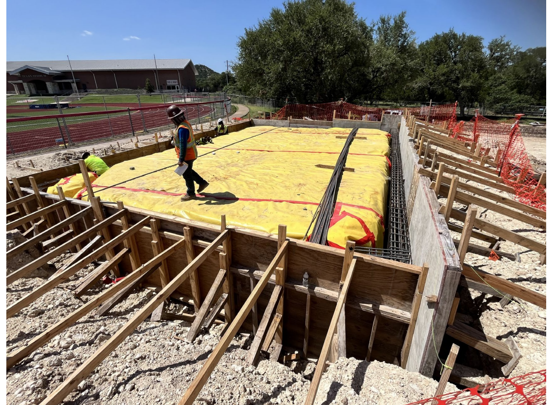
Photo: Track Storage Slab Prep
