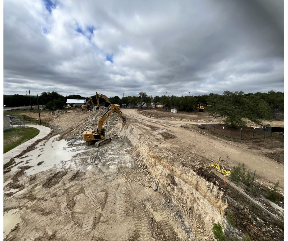
Photo: Band Marching Pad Retaining Wall
