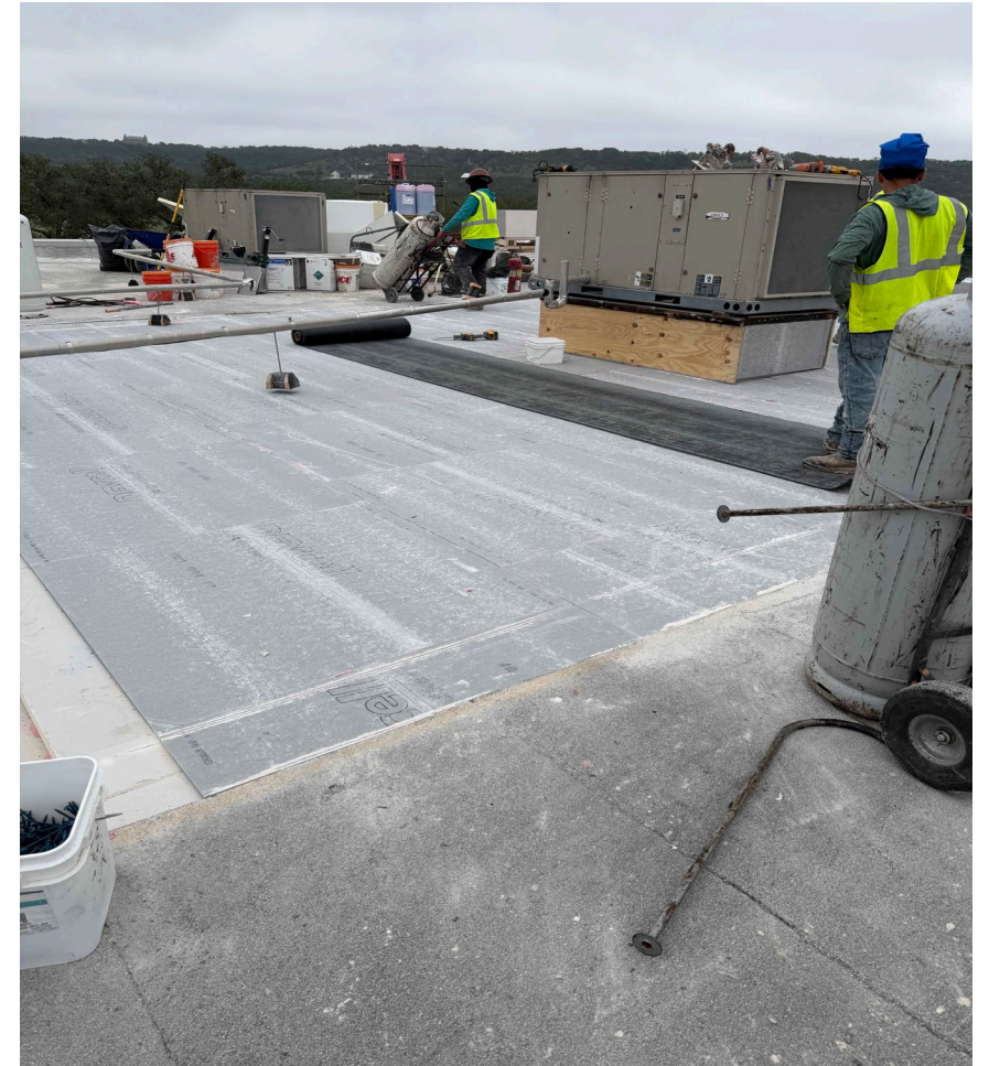
Photo: Roof replacement at Blue Hole
