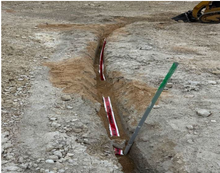
Photo: Marching Pad Electrical Trenching
