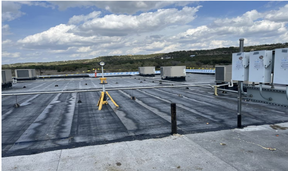
Photo: Roof Replacement at Blue Hole Primary
