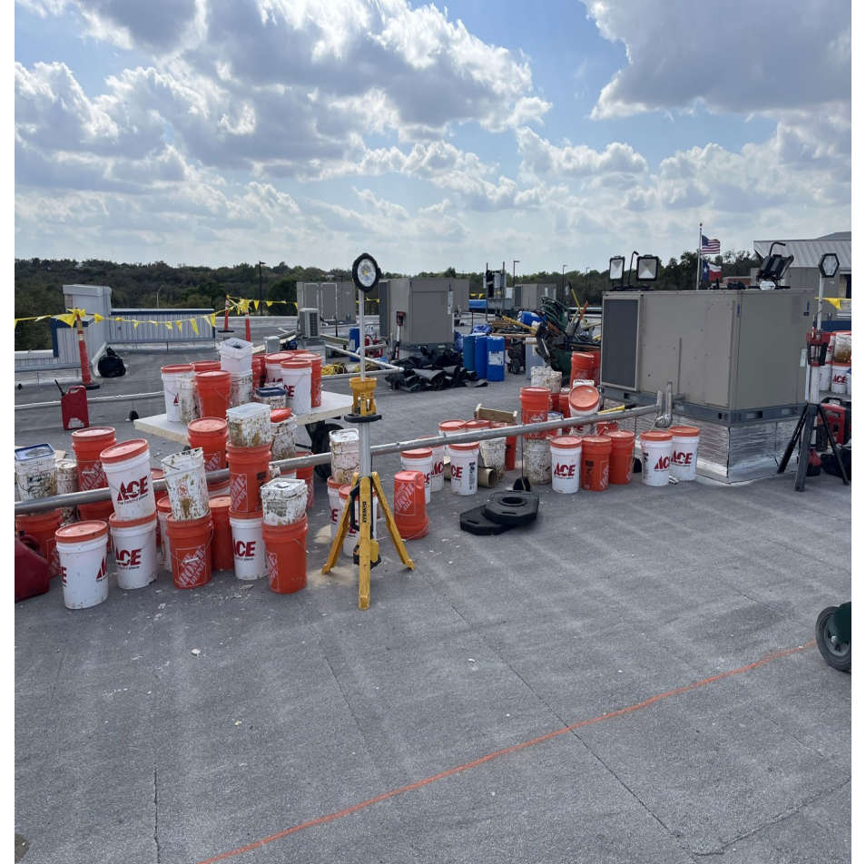
Photo: Roof Replacement at Blue Hole Primary
