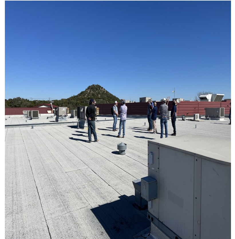
Photo: Roof at WHS
