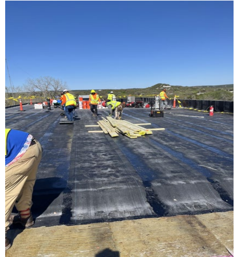
Photo: Roof replacement at Scudder
