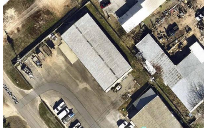
Network Operations Center
