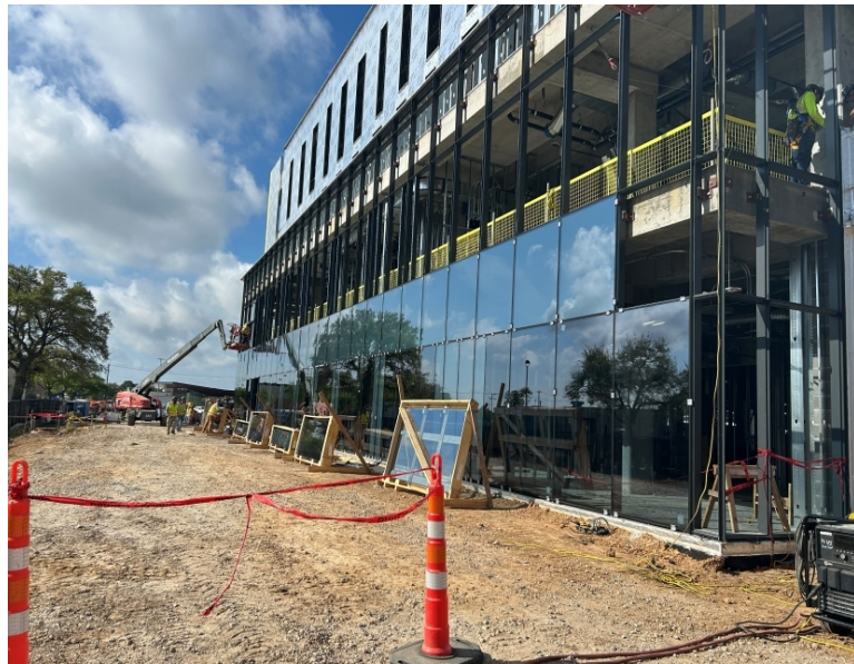
Exterior glazing in progress on the East elevation.
