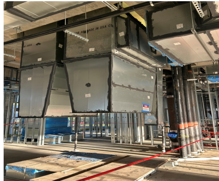
Overhead mechanical in progress throughout all floors.
