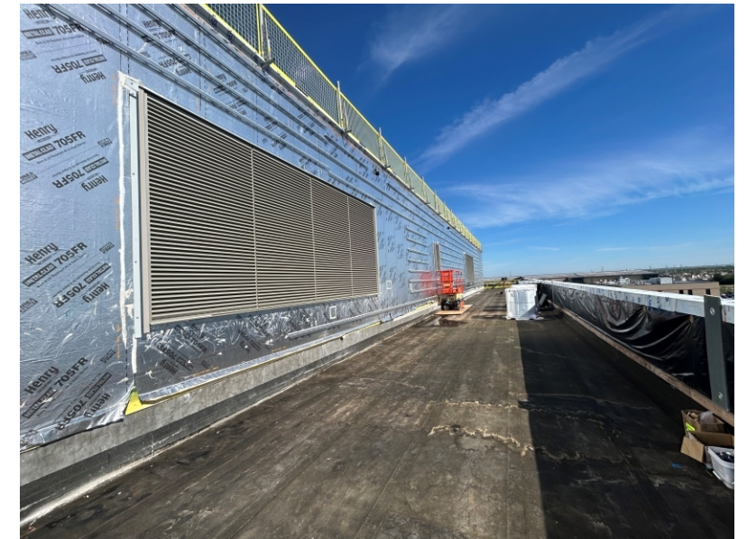
Penthouse louvers placed, metal panel installation in progress.
