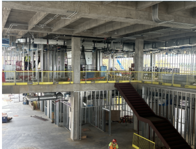
Overhead mechanical, electrical and plumbing- Lobby
