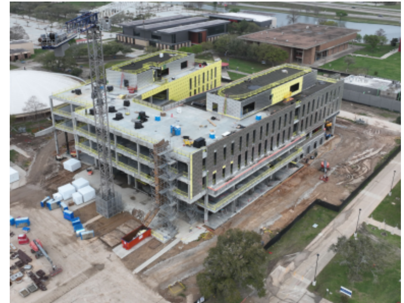
View from the southeast.
