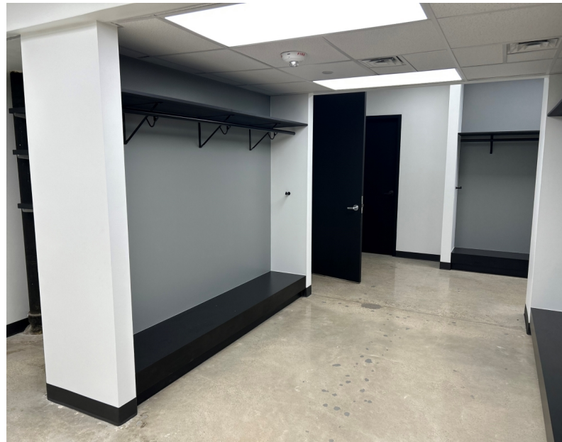
New finishes in progress at wardrobe area.
