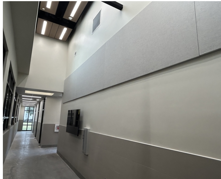
Welding Addition – main corridor
