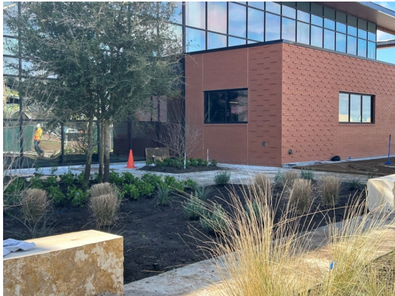
Landscaping in progress
