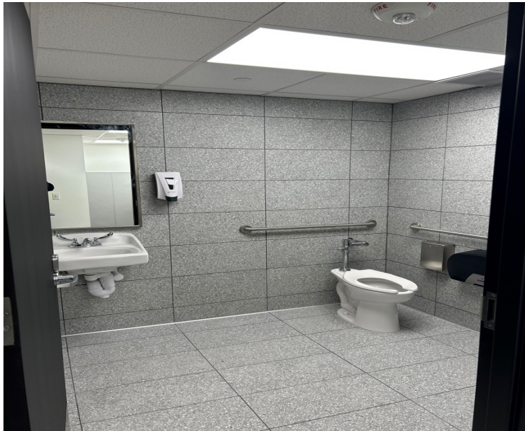
New restroom finishes.
