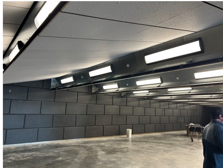
Shooting Range equipment installation
