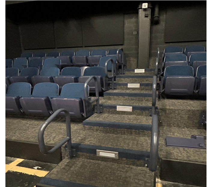
New theater seating in progress
