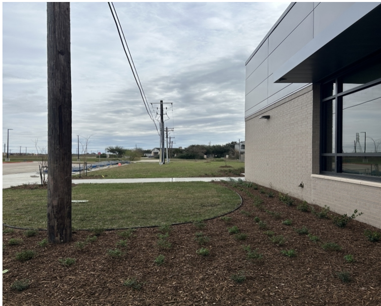
Welding Addition - Landscape
