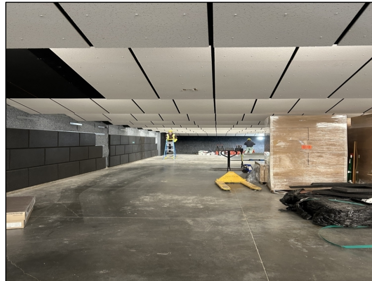
Shooting Range equipment installation
