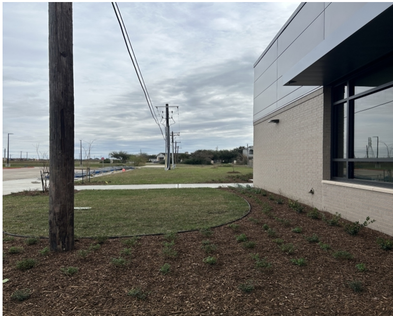
Welding Addition - Landscape
