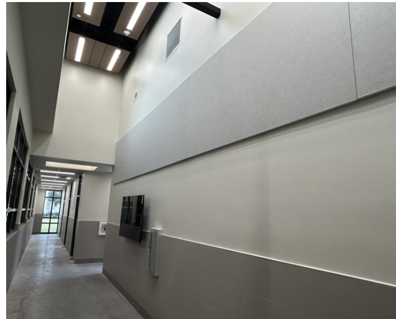
Welding Addition – main corridor
