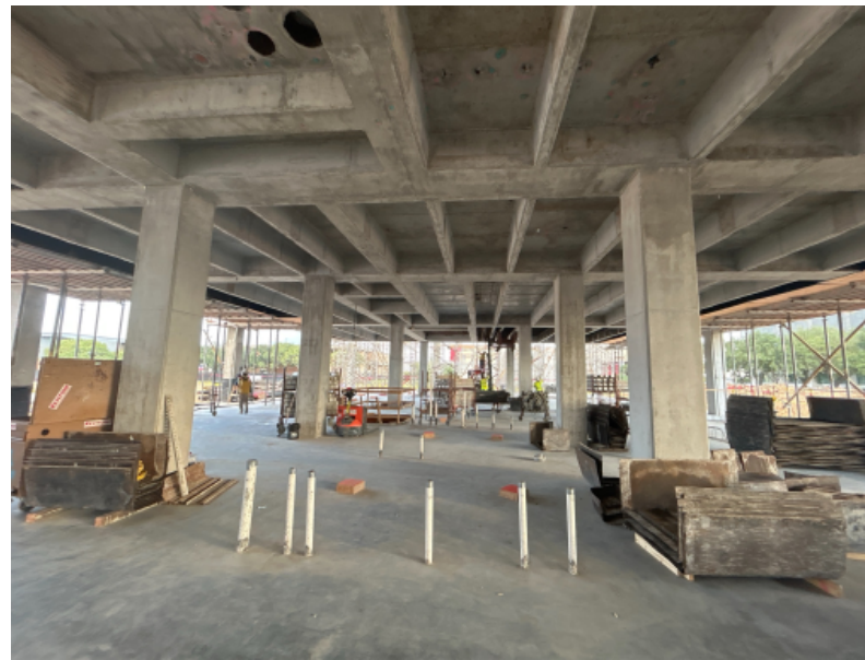
Shoring removed from Area A Second Floor Deck
