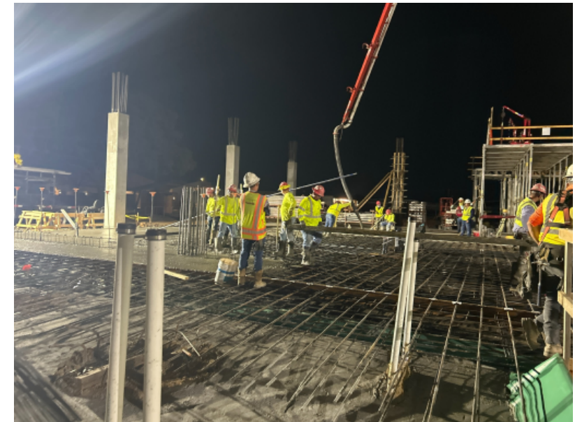
Slab-on-grade – Area C
