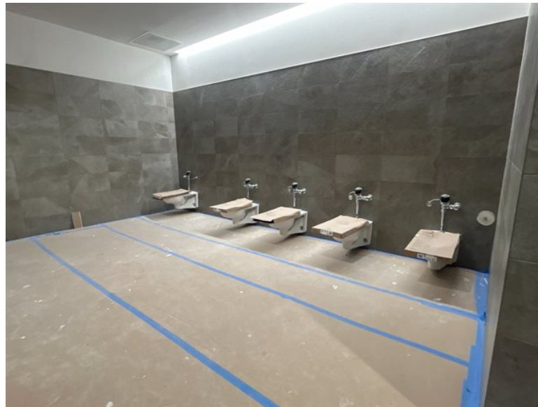
Restroom wall tile and fixtures
