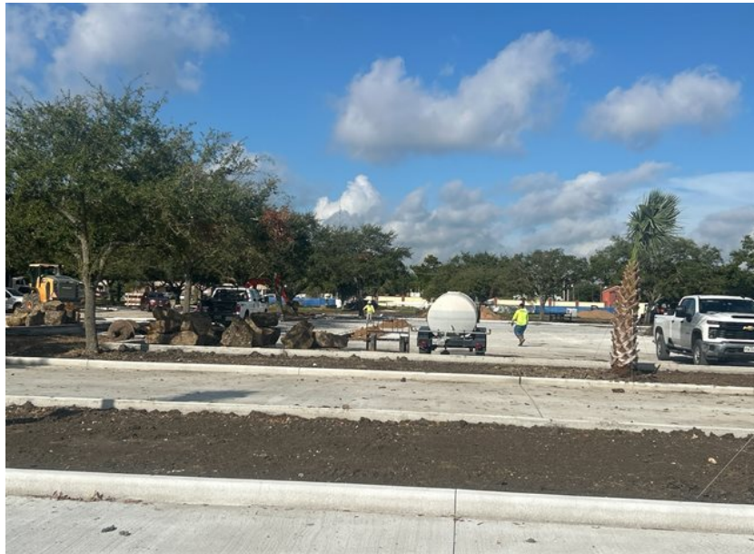
Landscaping at Lot A in Progress
