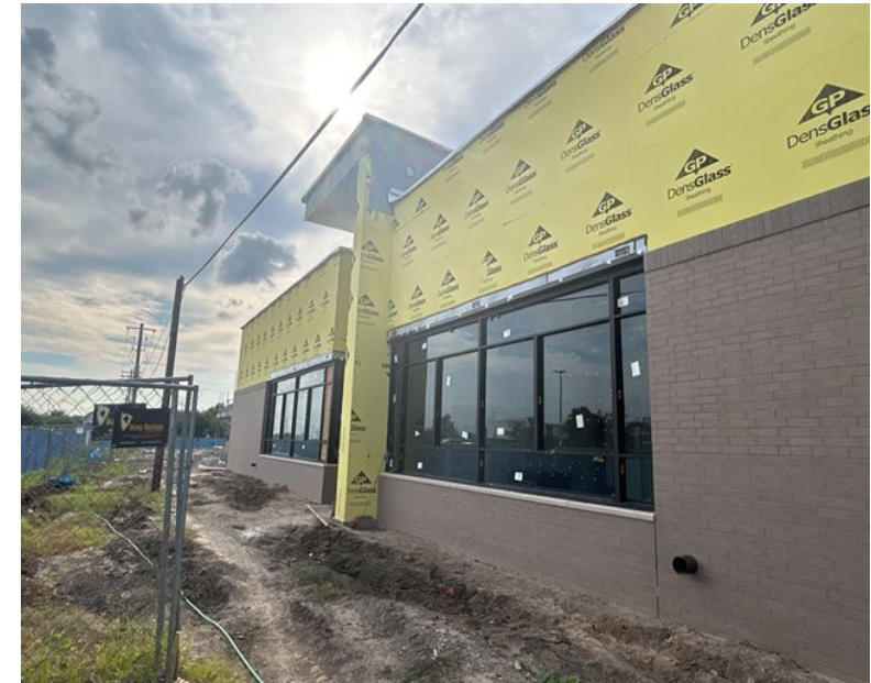
Welding Addition – Exterior brick and windows.
