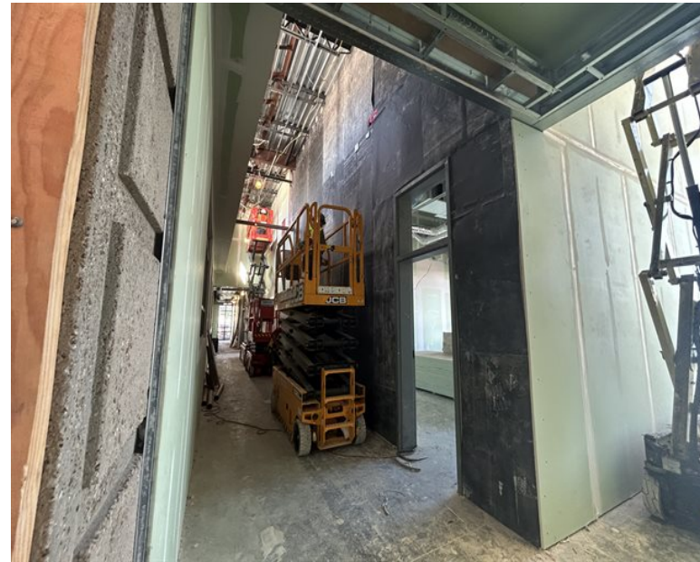
Welding Addition – drywall
