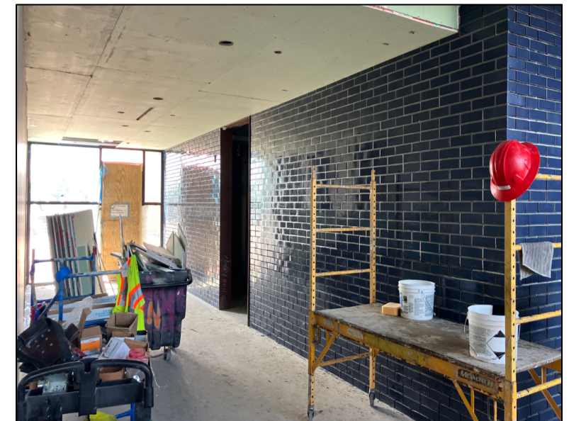
Wall tile – Area A
