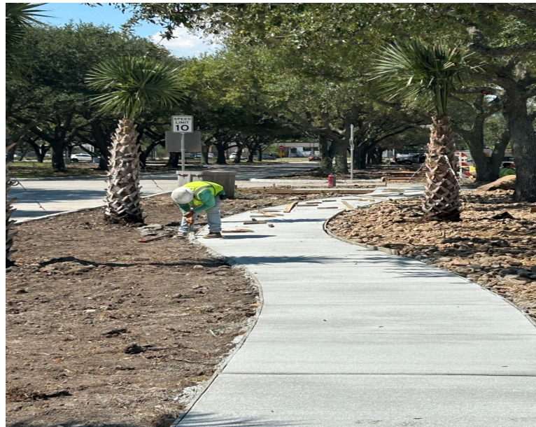
Sidewalks and ramps in progress at Lot A
