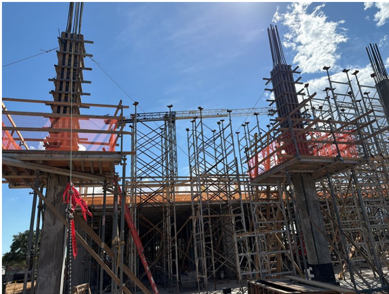
Elevated deck – Area A
