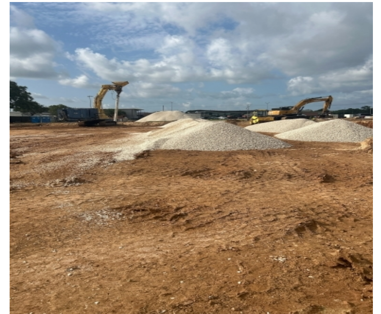
Stone column piers in progress
