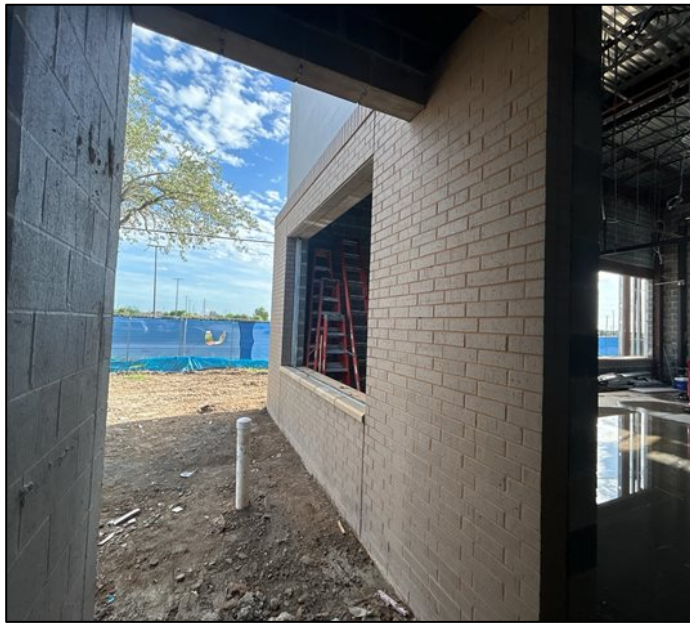
Brick complete at Welding Building Addition
