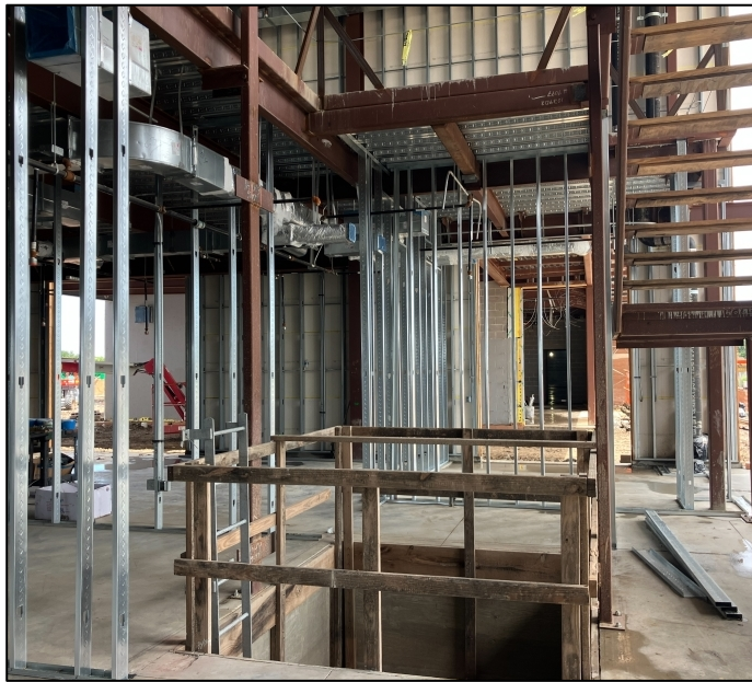
Interior framing at Area A
