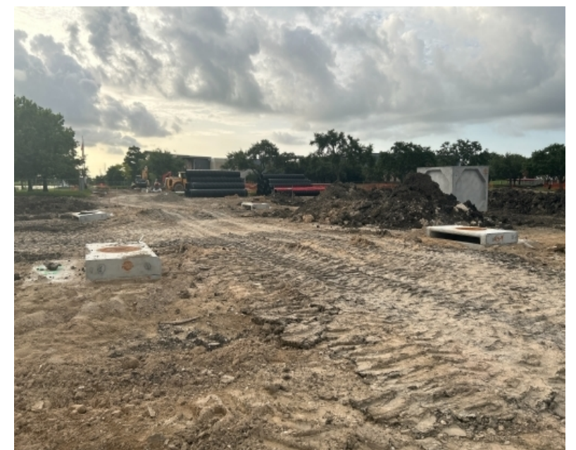
Storm drain pipe in progress at Lot A
