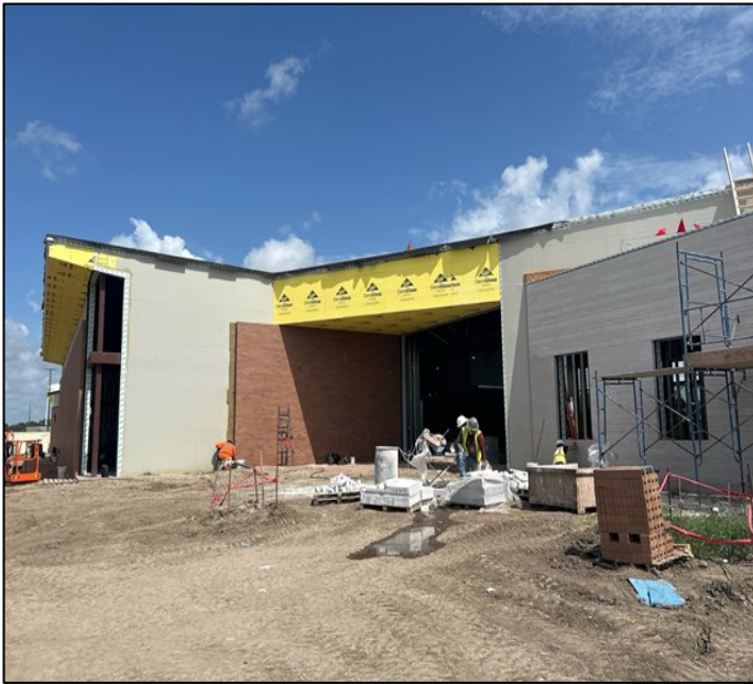
Masonry along front of building
