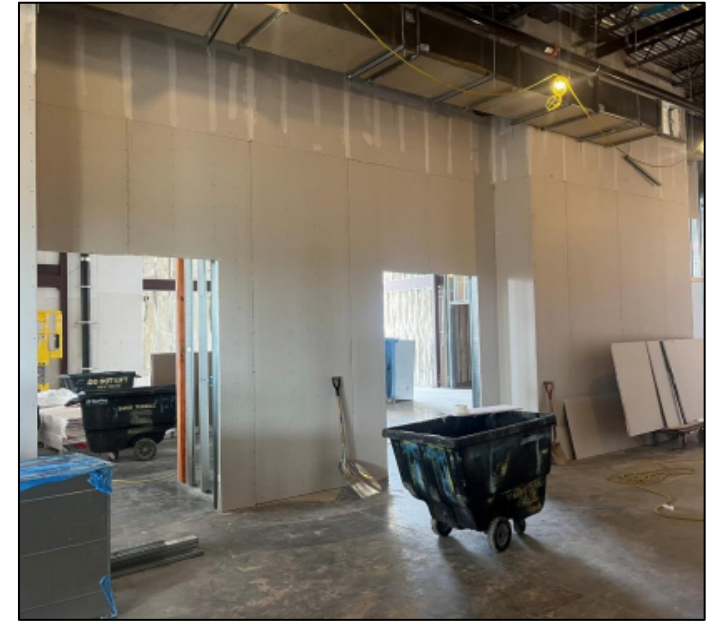
Drywall installation ongoing
