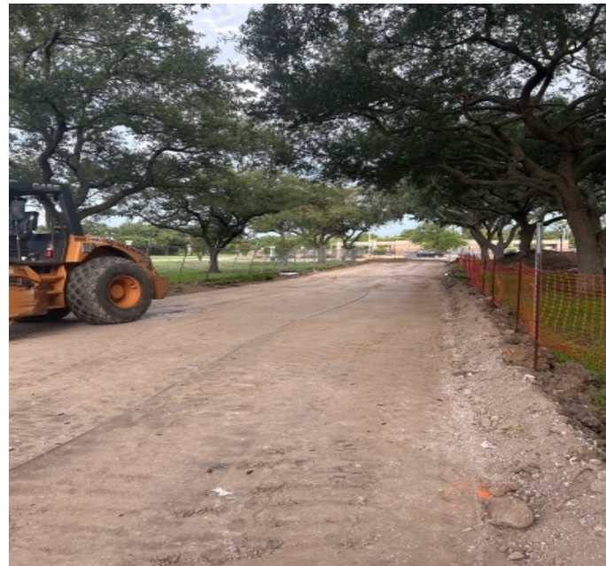
Fred Taylor Drive graded and ready for concrete crew
