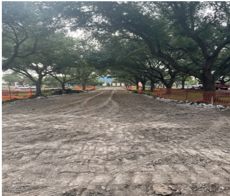
Fred Taylor Drive stabilized mixed base materials complete
