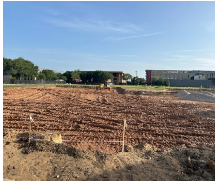
Engineered backfill near completion
