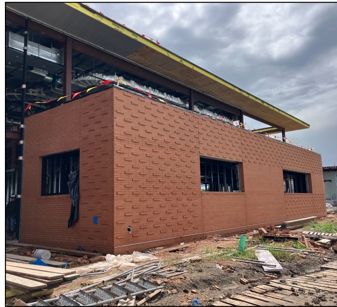
Brick work at Area A
