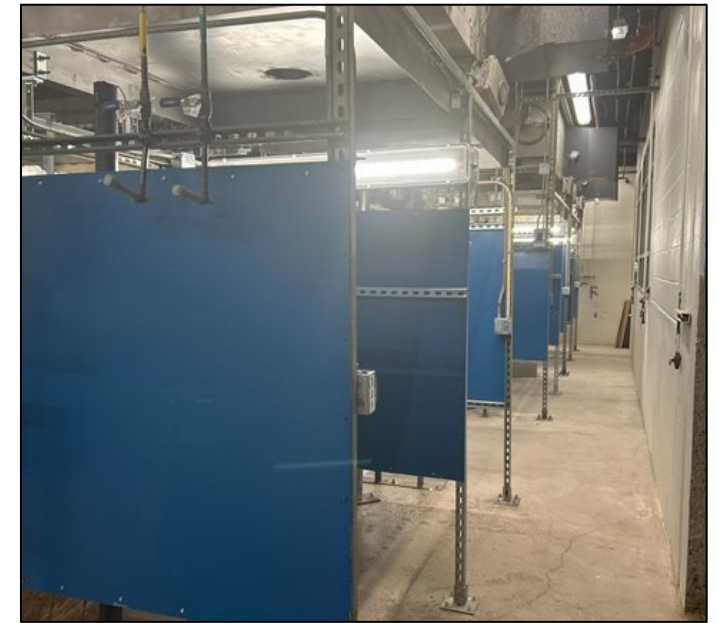
Renovated welding booths
