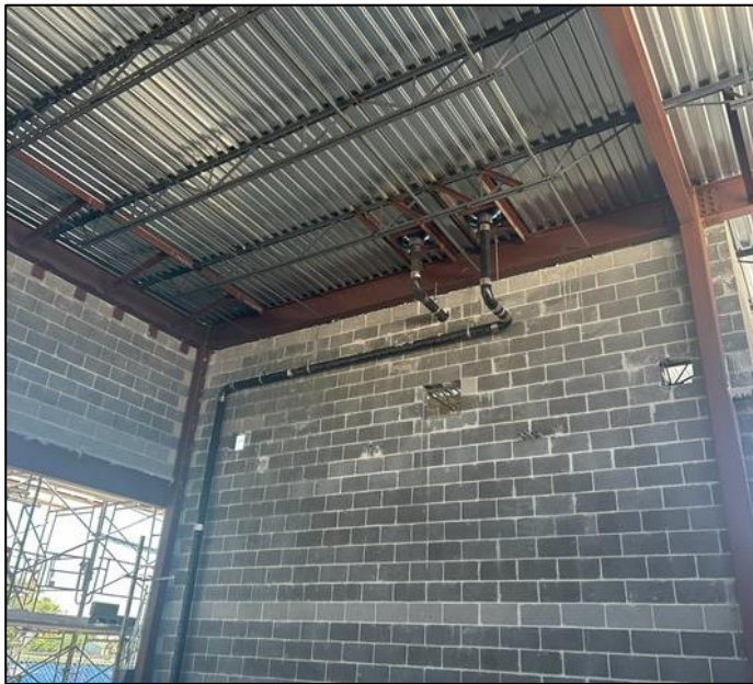
Masonry walls at Welding Building Addition
