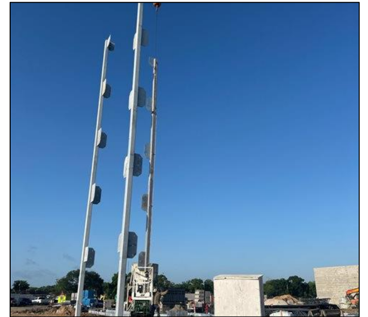
Training Tower structural steel
