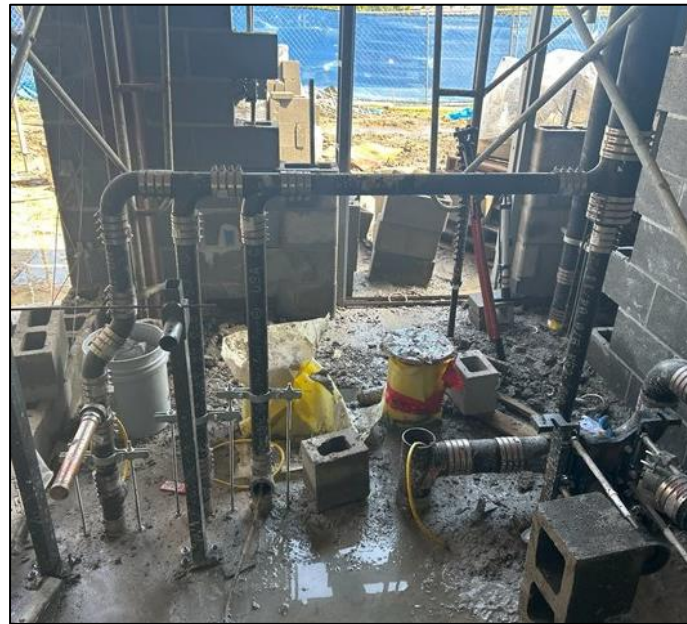
Plumbing for Welding Building Addition
