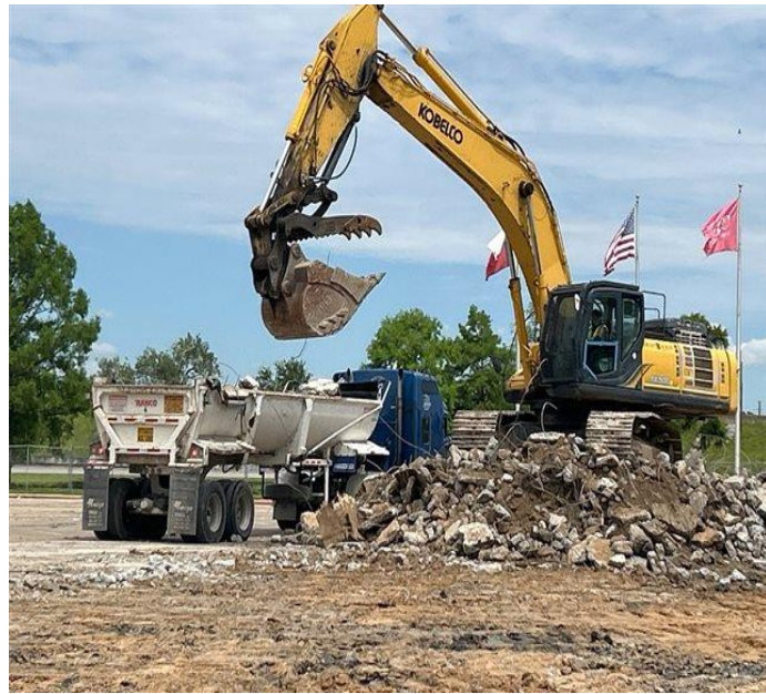
Demolition – Lot A
