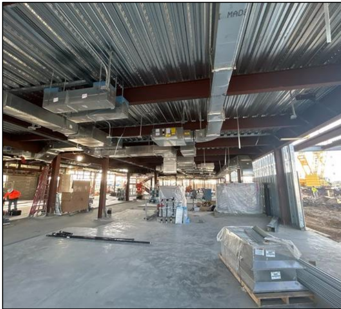
Overhead Mechanical Work
