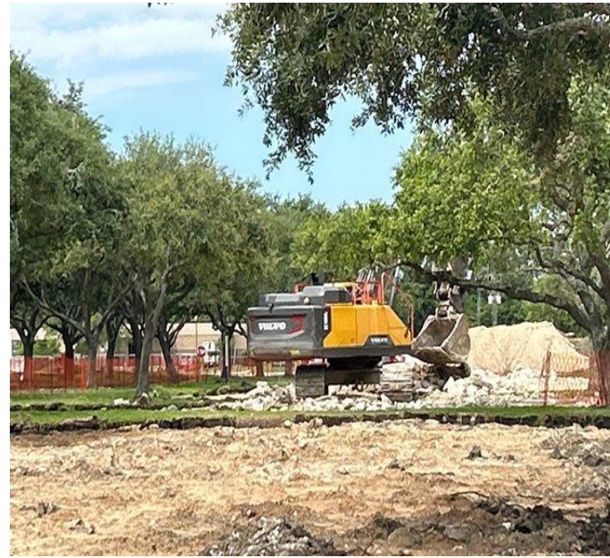
Demolition – Fred Taylor
