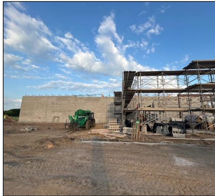
Masonry Walls at Shooting Range
