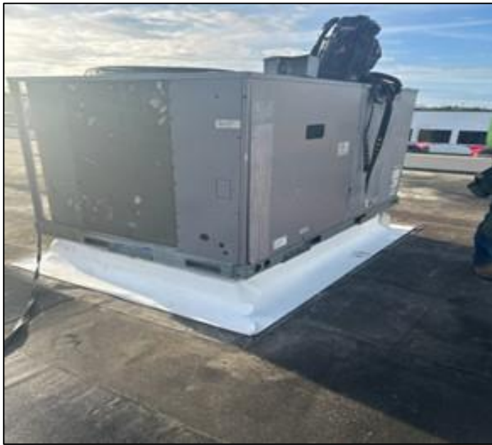
New Roofing Welding Building
