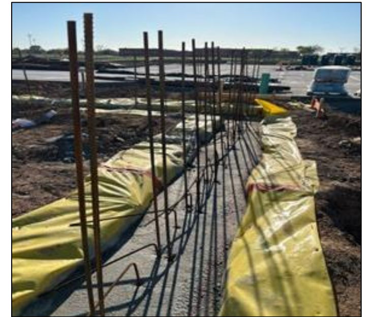
Grade Beam Footing at Firing Range Building
