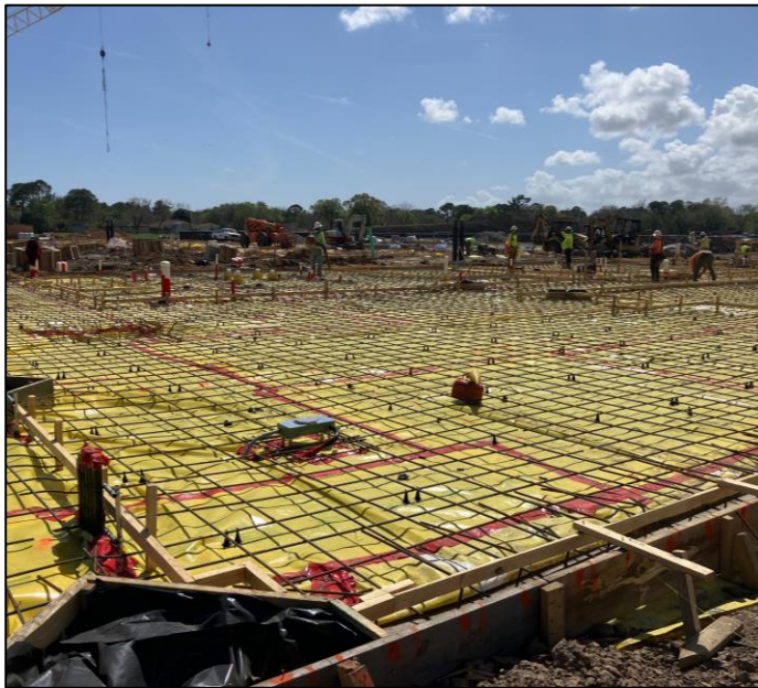
Forms and rebar for building slab
