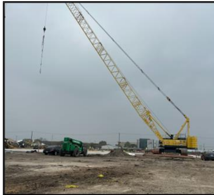
Crane delivery and set up
