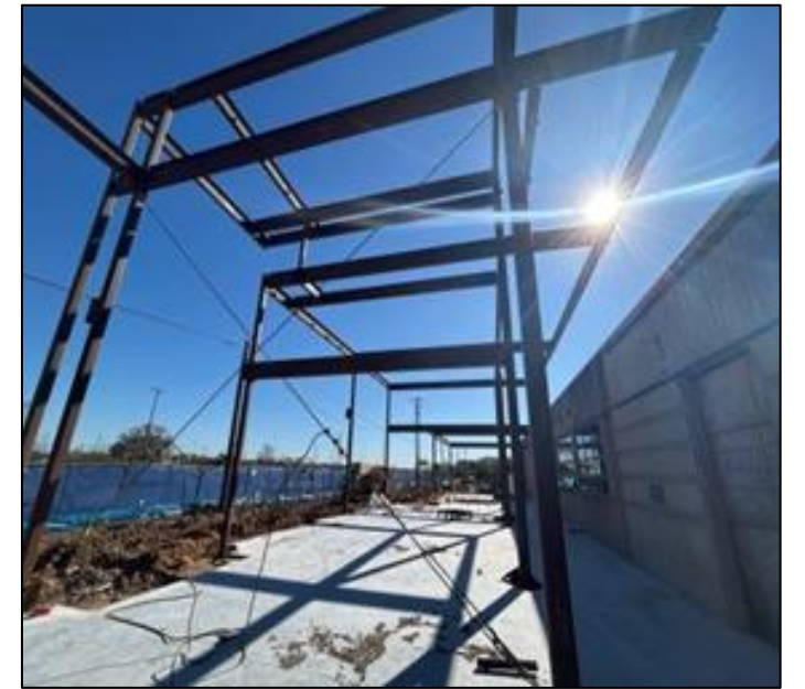
Structural Steel In Progress
