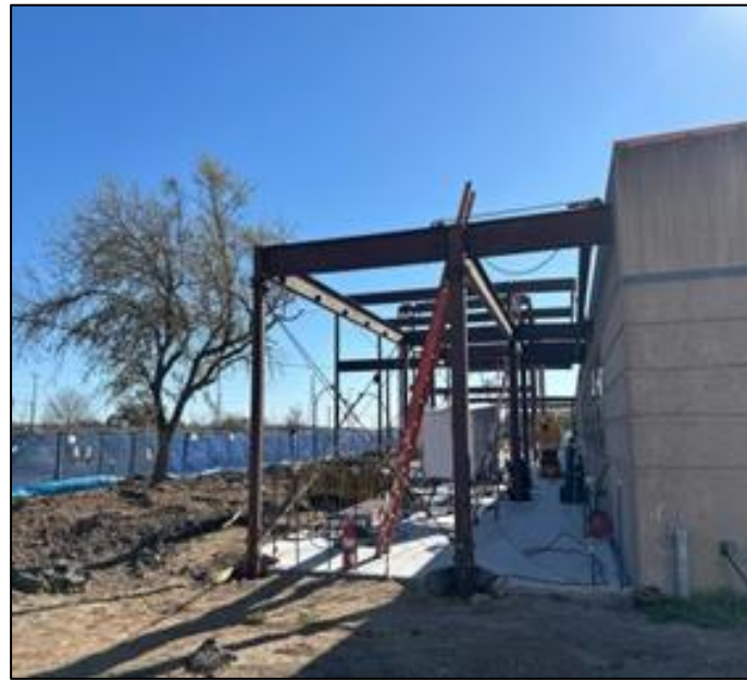
Welding Addition Structural Steel Installation
