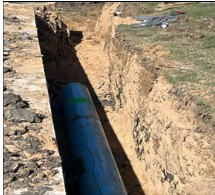
New 12" Water Line Service
