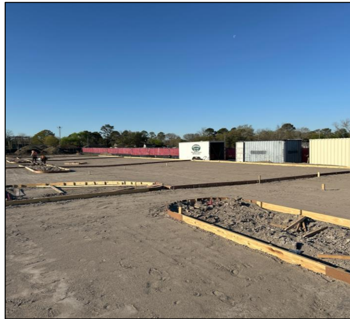
Concrete forms at Parking Lot
