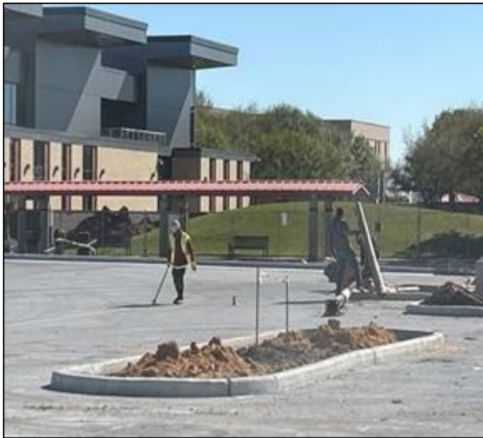
Caulking - Parking Lot B
