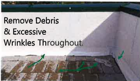
5. Typical, remove debris & wrinkles.
