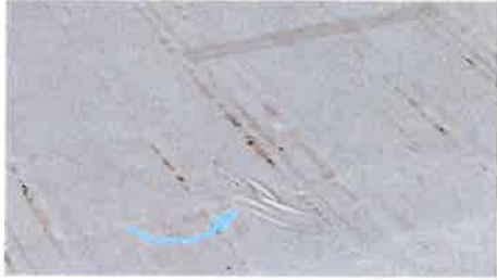
7. Typical; remove excessive wrinkles in field.
