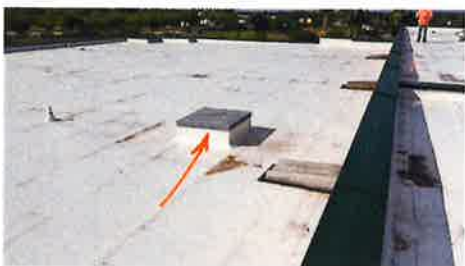
14. Typical, install proper sized caps on curbs.
