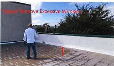
6. Typical, remove debris & wrinkles in flashing.
