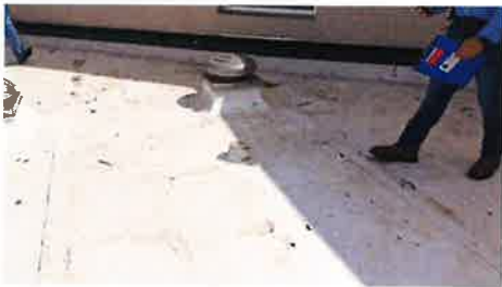
12. Typical, extend height of pipe penetrations.
