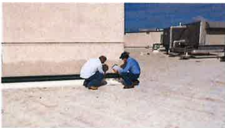
22. Typical, touch up stucco where needed.
