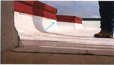
21. Typical, trim or extend corner flashing.
