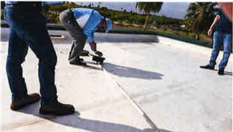
9. Typical, install & secure pads beneath pipe supports.
