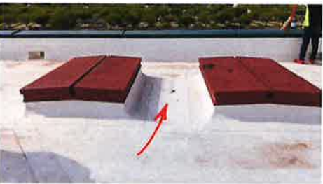
25. Typical, remove stains from surface of membrane.
