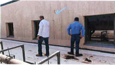
24. Typical, remove stains from walls.
