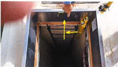
10. Relocate ladder up post to center of hatch.
