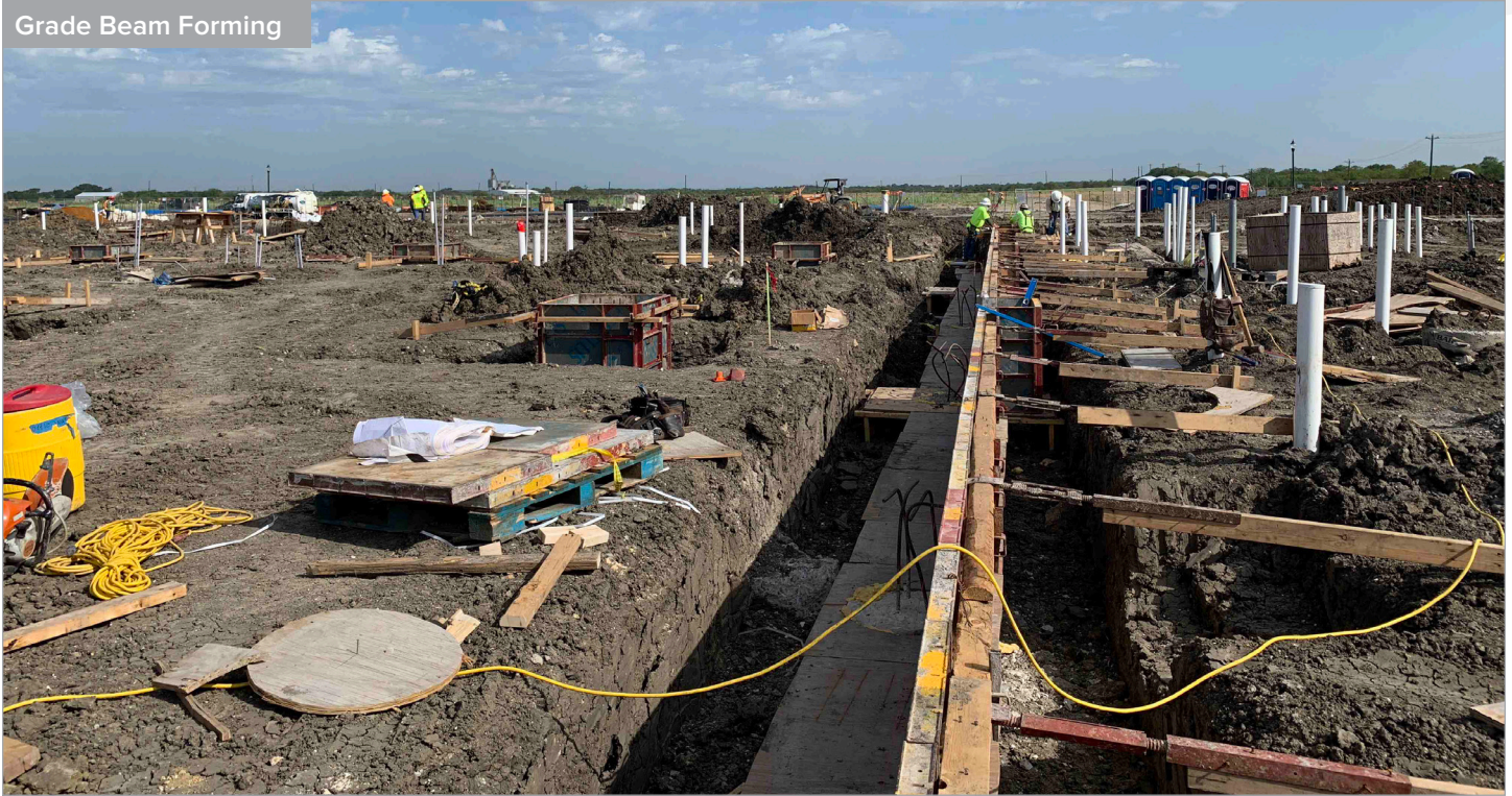
Grade Beams at Cafetorium Corridor
