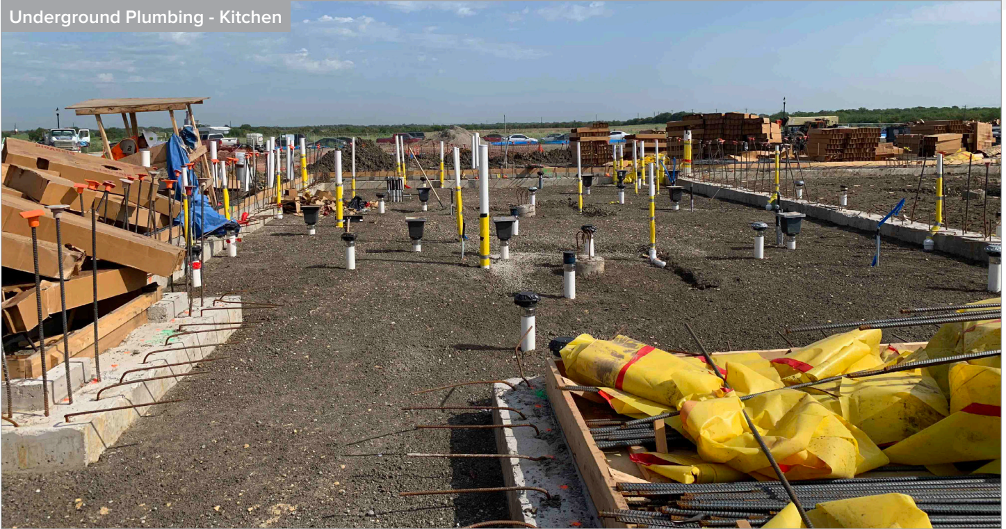
Placing of Pier Caps
