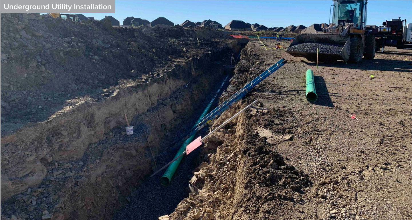
Underground Utility Installation
