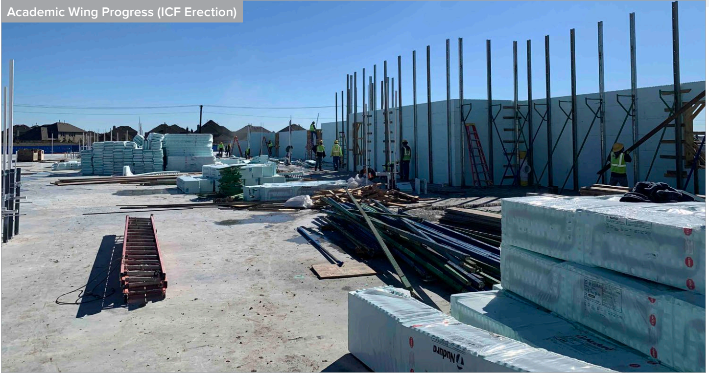
Close Up of ICF Construction
