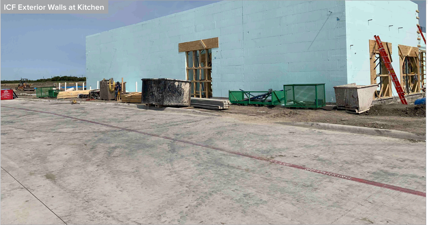
ICF Wall Erection and Bracing
