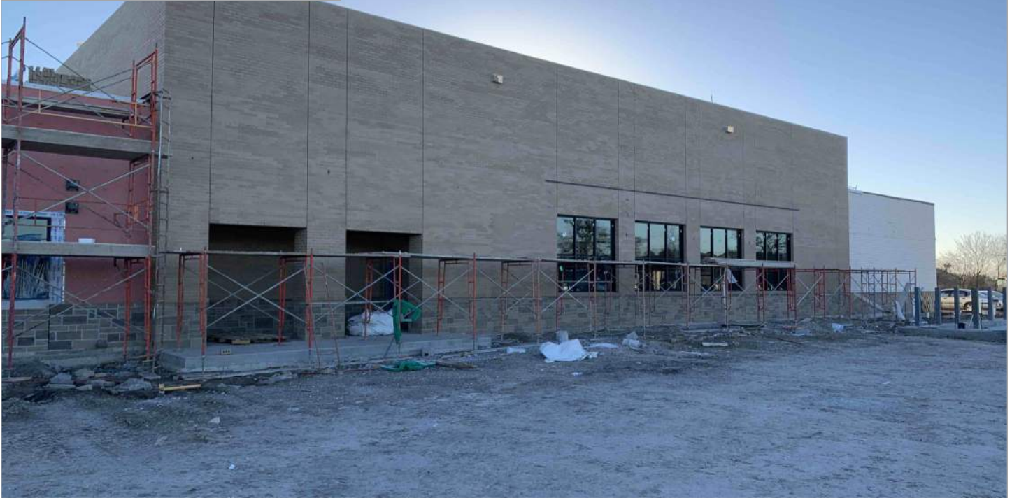
Exterior Masonry Veneer (Cafertorium)
