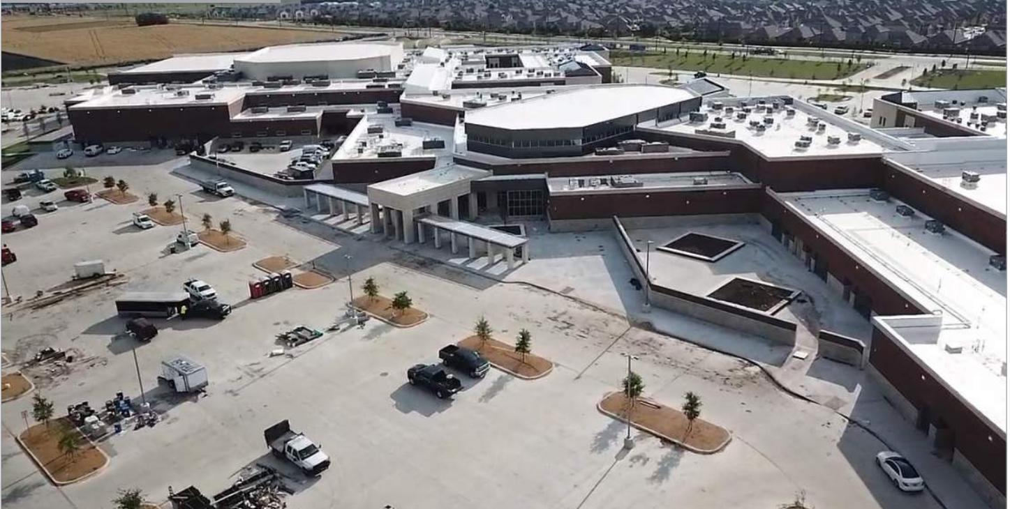
Aerial - Rear Looking Northeast
