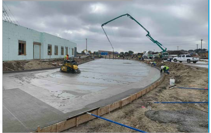
Concrete Fire Lane Placement
