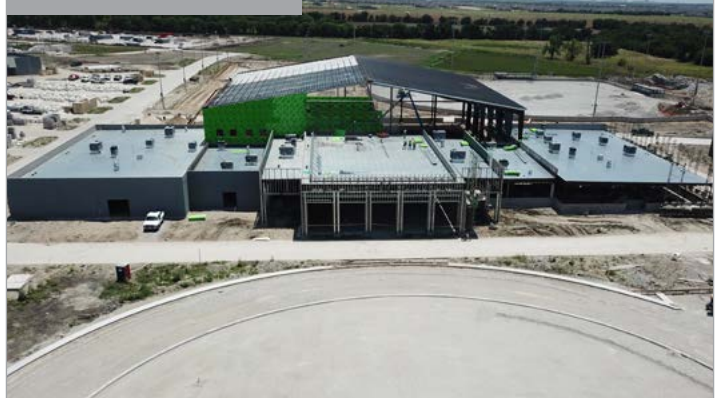
Aerial - MPF Building
