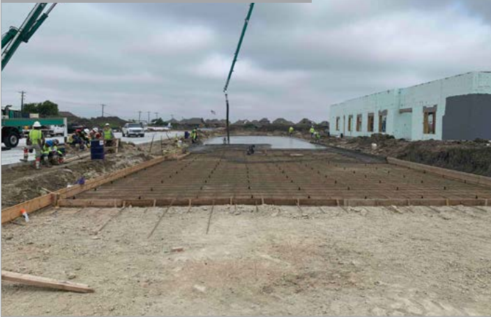
Concrete Fire Lane Placement
