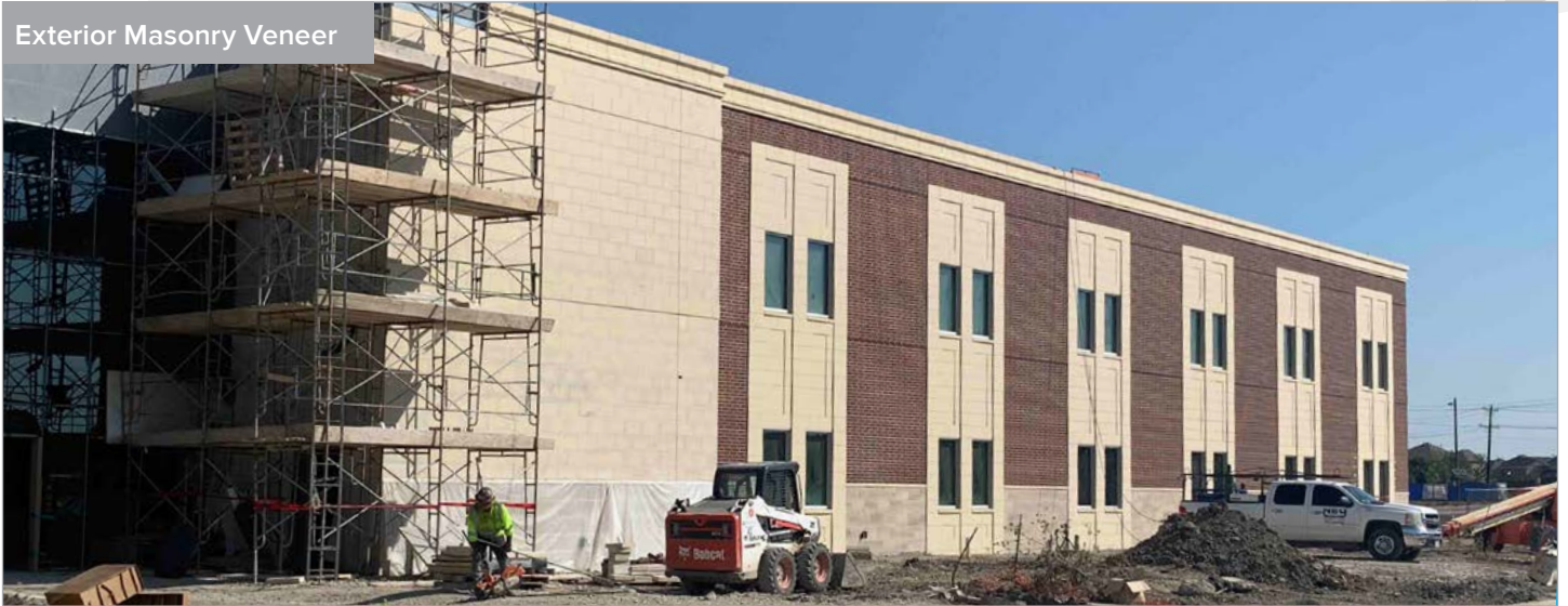
Indoor Practice Facility
