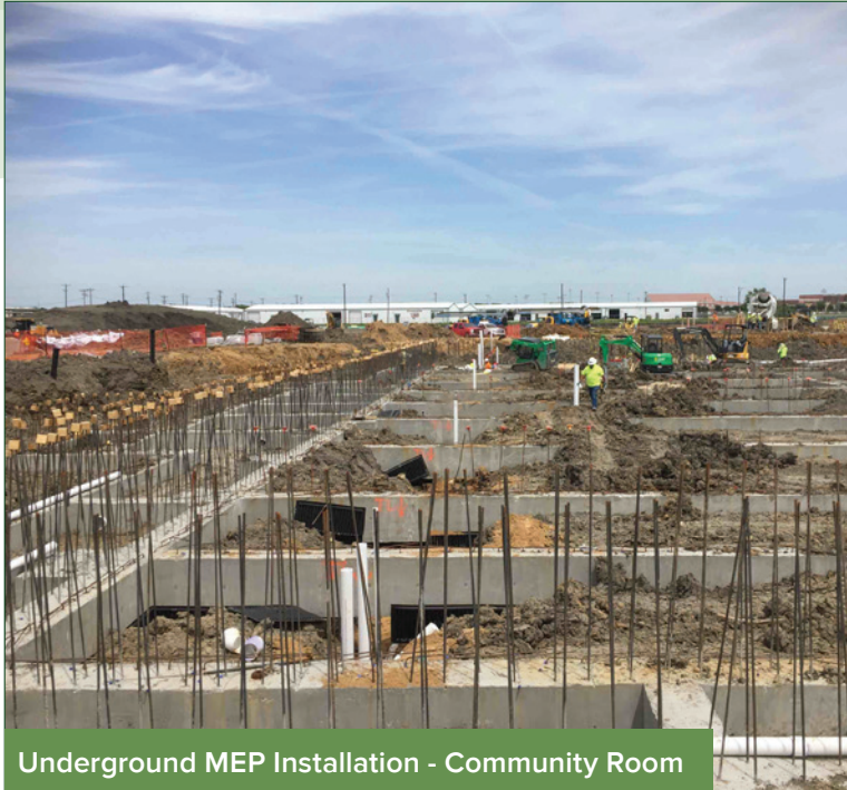
Installation of Electrical Underground
