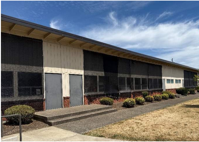
1. South façade classrooms with temporary shading devices to try to keep rooms cooler.
