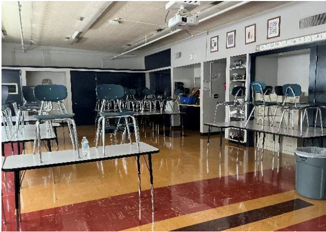
1. Original classrooms with ACM flooring and fluorescent lighting.
