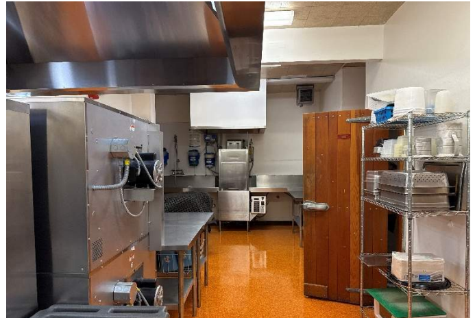
4. Aged kitchen equipment in an undersized space.
