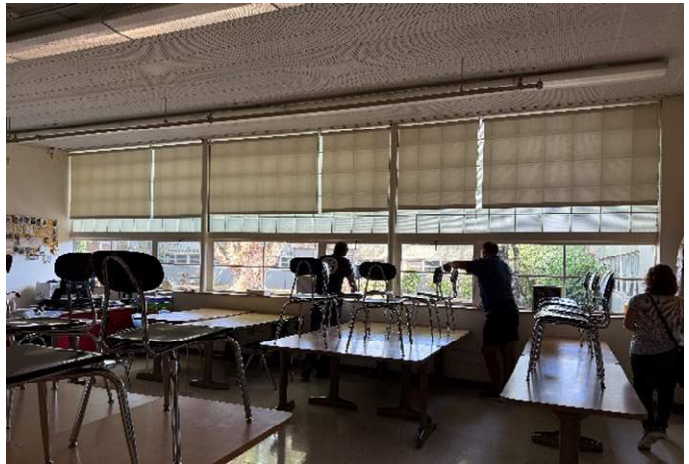
4. Original single-pane windows.
