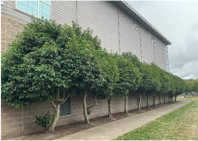
3. Trees planted too close to building.
