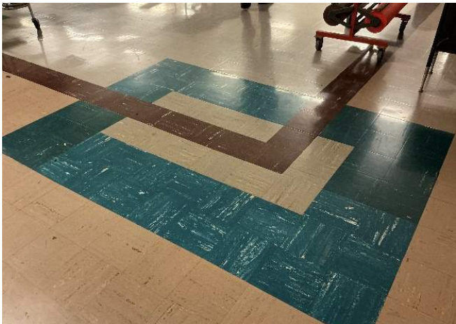
3. ACM Flooring in Cafeteria.
