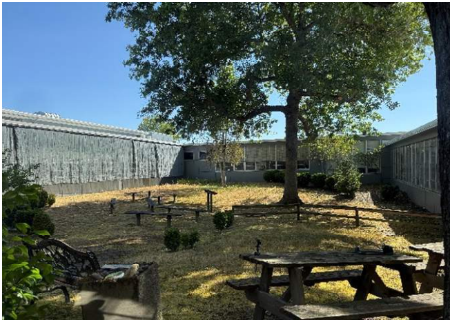
3. Shade fabric over windows to reduce heat gain.
