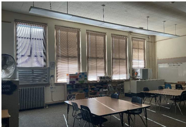
5. Third floor classroom, added unit ventilator and fluorescent lighting.
