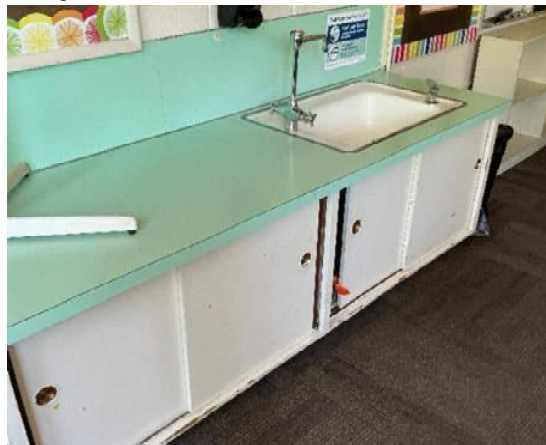
6. Original casework and plumbing fixtures in classroom.
