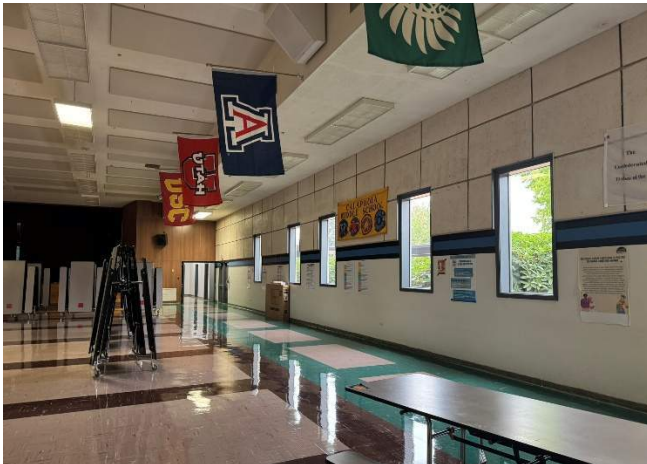
9. Presumed ACM flooring in the cafeteria, fluorescent lighting fixtures.
