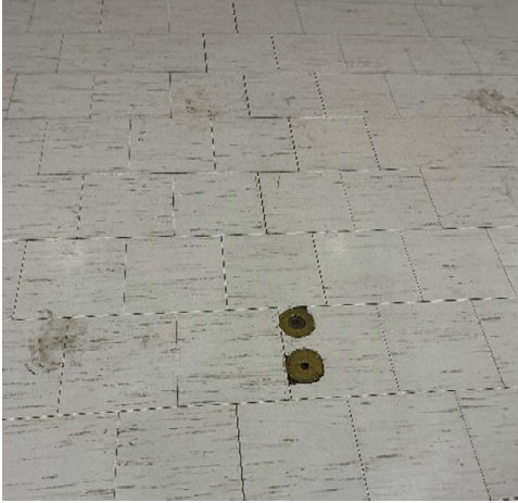
7. ACM Flooring in cafeteria.
