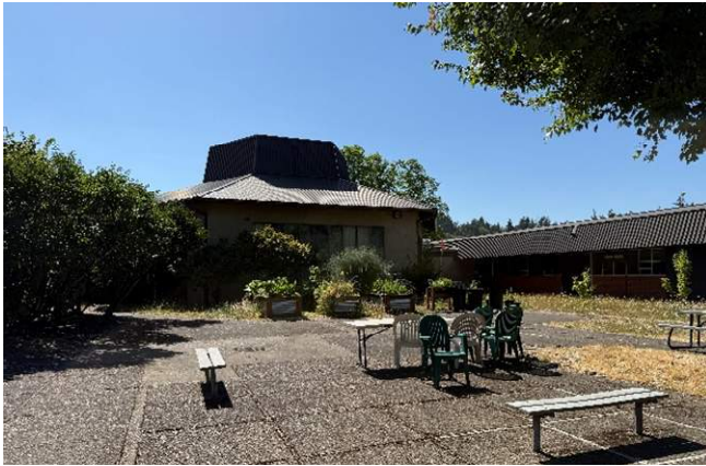
3. Center courtyard has limited access and drainage issues. All paving and grading should be redone.
