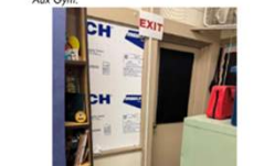
4. Exterior exit in classroom, missing illuminated signage, temporary insulation visible to help regulate temperature in room.
