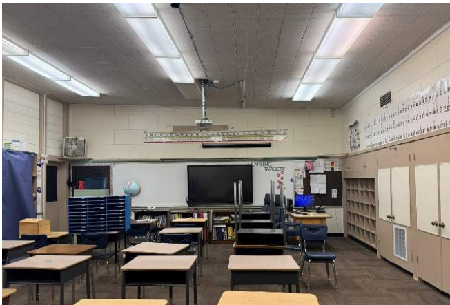
7. Typical classroom, original casework, fluorescent lighting, painted block at exterior wall.
