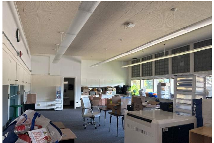
6. Typical classroom in original building, fluorescent lighting and original casework.
