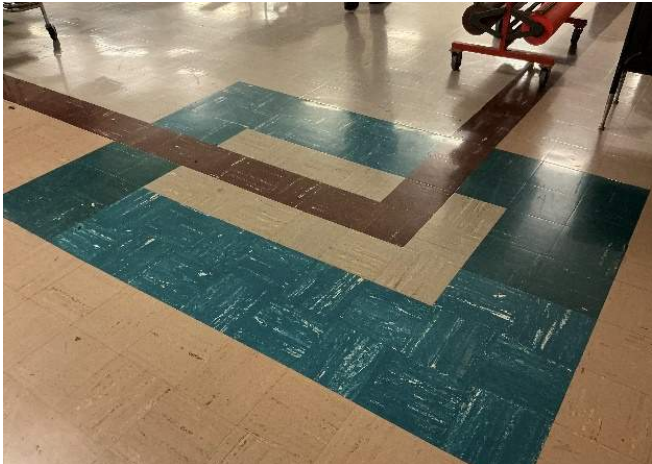
3. ACM Flooring in Cafeteria.
