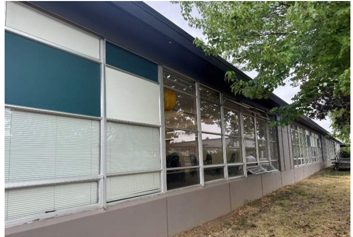
8. Typical exterior aluminum framed windows.
