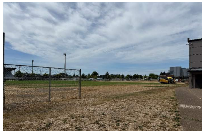
6. Playfield condition is poor and walking track has been overgrown.
