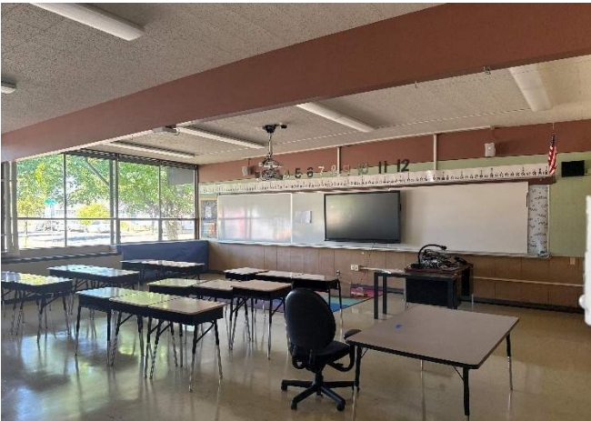
5. Typical classroom in addition, fluorescent lighting, presumed ACM flooring.
