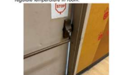
6. Visible gap in exterior door at Aux Gym
