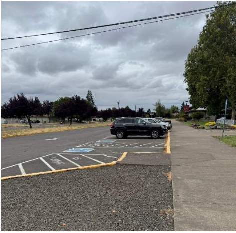
1. ADA Parking and paving needs to be updated.
