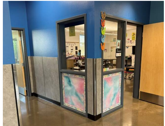
6. Teacher's temporary modification of the interior glazing.
