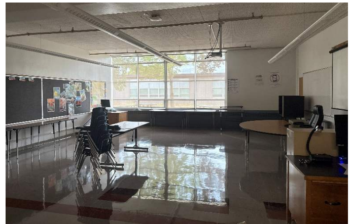
10. Classroom, updated lighting and wall finishes, but presumed ACM flooring remains.
