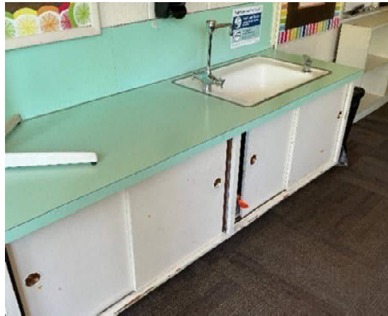
6. Original casework and plumbing fixtures in classroom.
