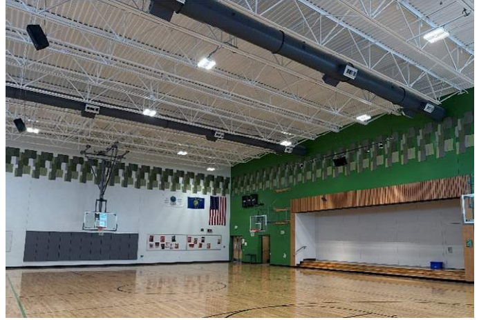
2. Despite acoustic treatment on walls, noise is a consistent issue for using the gym.
