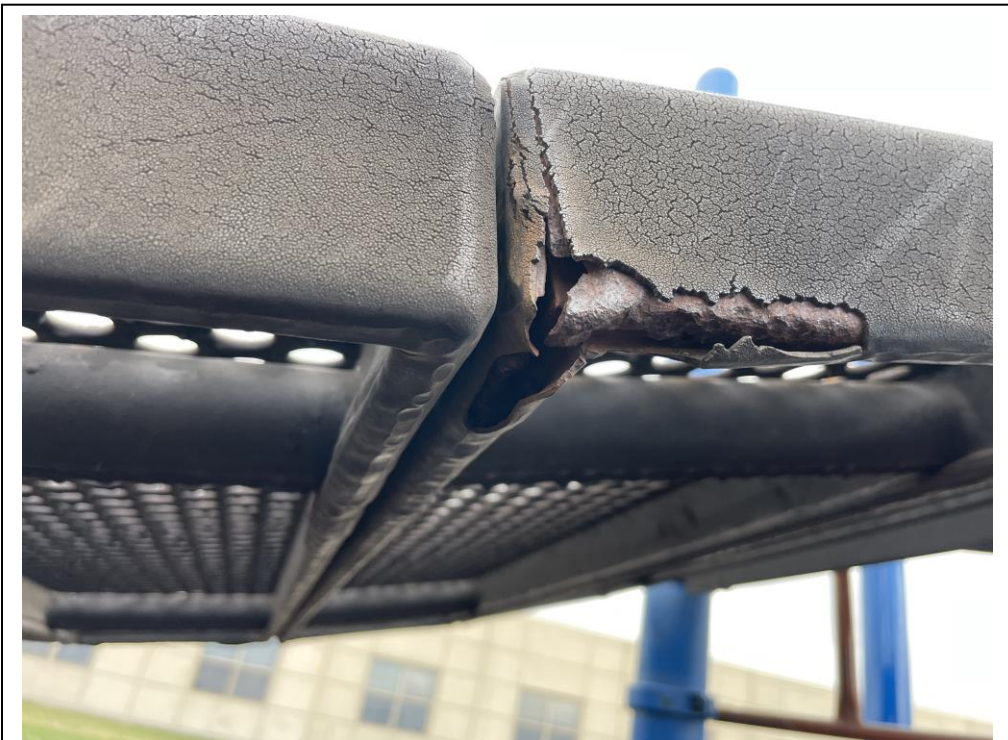
Close-up image of deterioration and sharp rusty edges.
