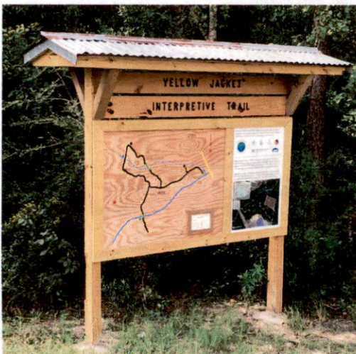
Two new entry kiosks were designed by GCCDS and LaTerre Bioregional Center. GCCDS coordinated the construction process with students, faculty, and community members.
