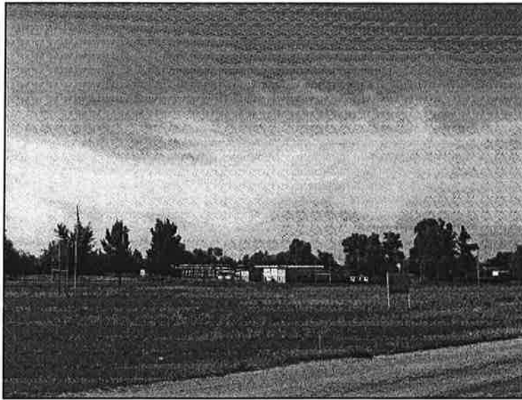
2675 Northwest Loop Overall View of Subject Looking Southwest
