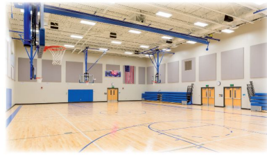
New Gym addition with restrooms
